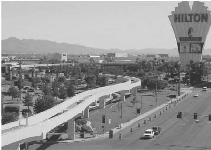
Las Vegas Monorail - 2004 Excellence in Concrete
