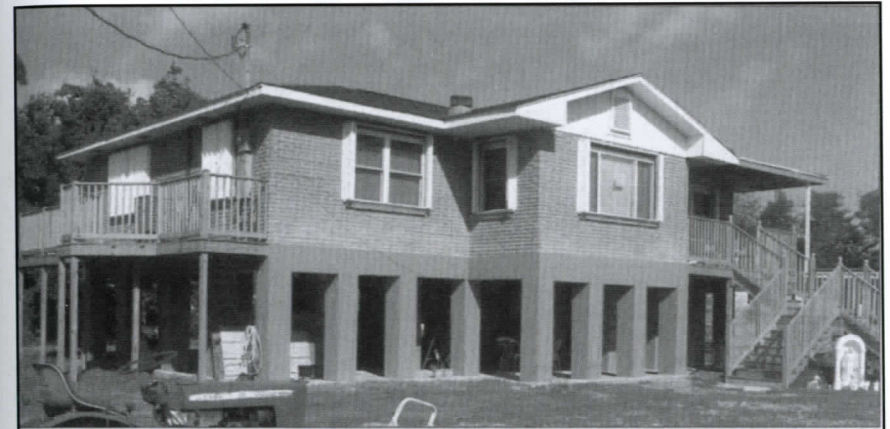
FRONT AND LEFT SIDE COLUMNS AND SLAB FORM ARCHES
