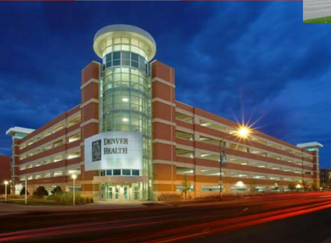
The Denver Health Employee Parking Garage provides 228,000 ft<sup>2</sup> of parking in five stories. The structure has an open interior created by double tees that span between “spread walls” and K-frames, which also resist lateral loads. Altogether, 927 pieces of architectural and structural precast products went into the building. The architectural concrete wall panels were cast with thin brick, and the surrounding colored concrete was lightly acid-etched.
