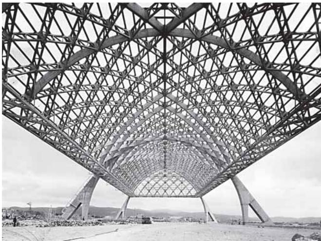
Pier Luigi Nervi's 1936 design of a hangar near Rome, Italy, had a lamella-type shell roof composed of precast reinforced concrete lattice members with only six supporting buttresses. The large ribs were solid, cast-in-place members.
