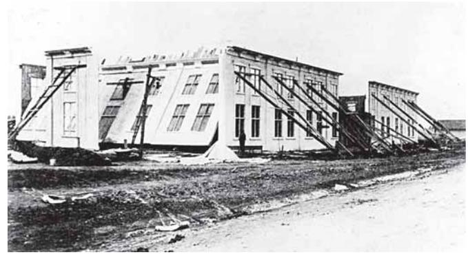
One of the earliest site-cast, tilt-up wall panel construction projects was undertaken circa 1907 by Robert Aiken at Camp Perry, OH. The wall was cast upon a large tipping table (left). After 48 h, when the concrete was solid, jacks tipped the wall into position, the wall was braced, and the platform moved to the next position.
