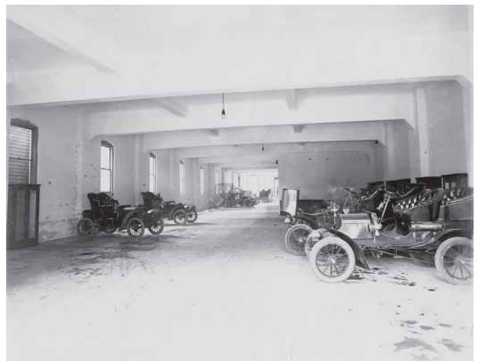
C. A. P. Turner was one of the pioneers in reinforced concrete construction in the U.S. He is credited as one of the inventors of the flat slab system and built the first flat slab, the Bovey-Johnson Building in Minneapolis, MN, on a 14 x 17 ft (4 x 5 m) module in 1906. Turner's system was used in this garage erected in the early 1900s.
