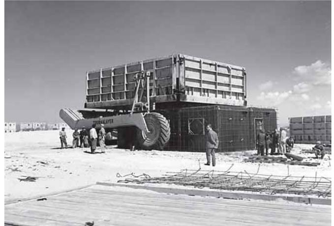
Thomas A. Edison developed a mass production system of building concrete houses in one-piece metal molds circa 1910. R. G. LeTourneau took the method to new heights in the 1940-1950 decade. One of the most notable attempts at large-scale concrete prefabrication of homes was the LeTourneau process invented in 1946. The house-molding machine was used to build a neighborhood in Longview, TX, in the late 1940s and later in Haifa, Israel, in the 1950s.
