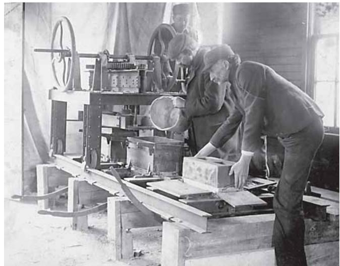
A circa 1900 concrete block manufacturing operation.
