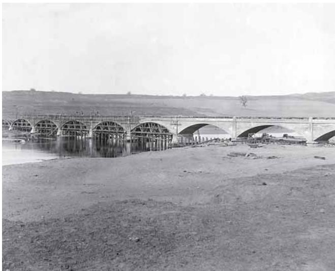
Concrete Bridge at Pollasky, Cal., Ten 75-foot Spans, Reinforced with Corrugated Bars, Designed by Jno. B. Leonard, C. E.
