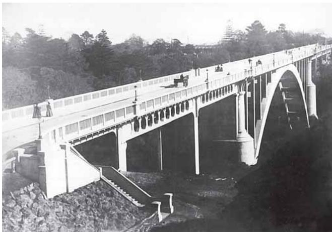
An outstanding early bridge: the Grafton Bridge, Auckland, New Zealand. Opened to traffic in 1910, the bridge was made up of one 42 ft (13 m) span, two spans 78.5 and 80.5 ft (24 and 25 m), a main arch span of 320 ft (98 m), four spans 75.5 ft (23 m) each, and two spans 35 and 37.5 ft (11 and 11.5 m). Design and construction by Ferro-Concrete Co. of Australia. *ACI archives. Photo courtesy of Auckland City Engineer's Office.*
