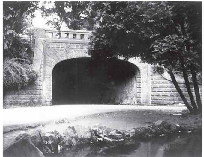
Alvord Bridge in San Francisco's Golden Gate Park was built in 1889 by Ernest L. Ransome. The reinforced concrete bridge is believed to be the oldest—and first to be constructed—concrete bridge with steel reinforcing bars in the U.S. The cold-twisted steel square reinforcing bar system was an invention of Ransome.
