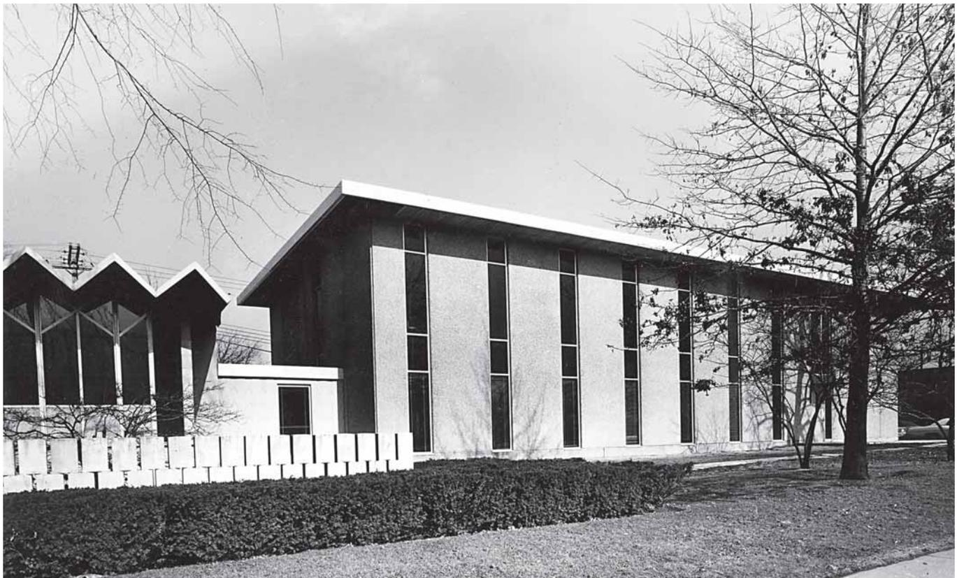
The Institute expanded the Detroit headquarters with the construction of a second building in 1969. The east building (right) featured reinforced concrete beam-and-column framing, faced with two-story exposed aggregate precast panels using Michigan crushed stone aggregate.
