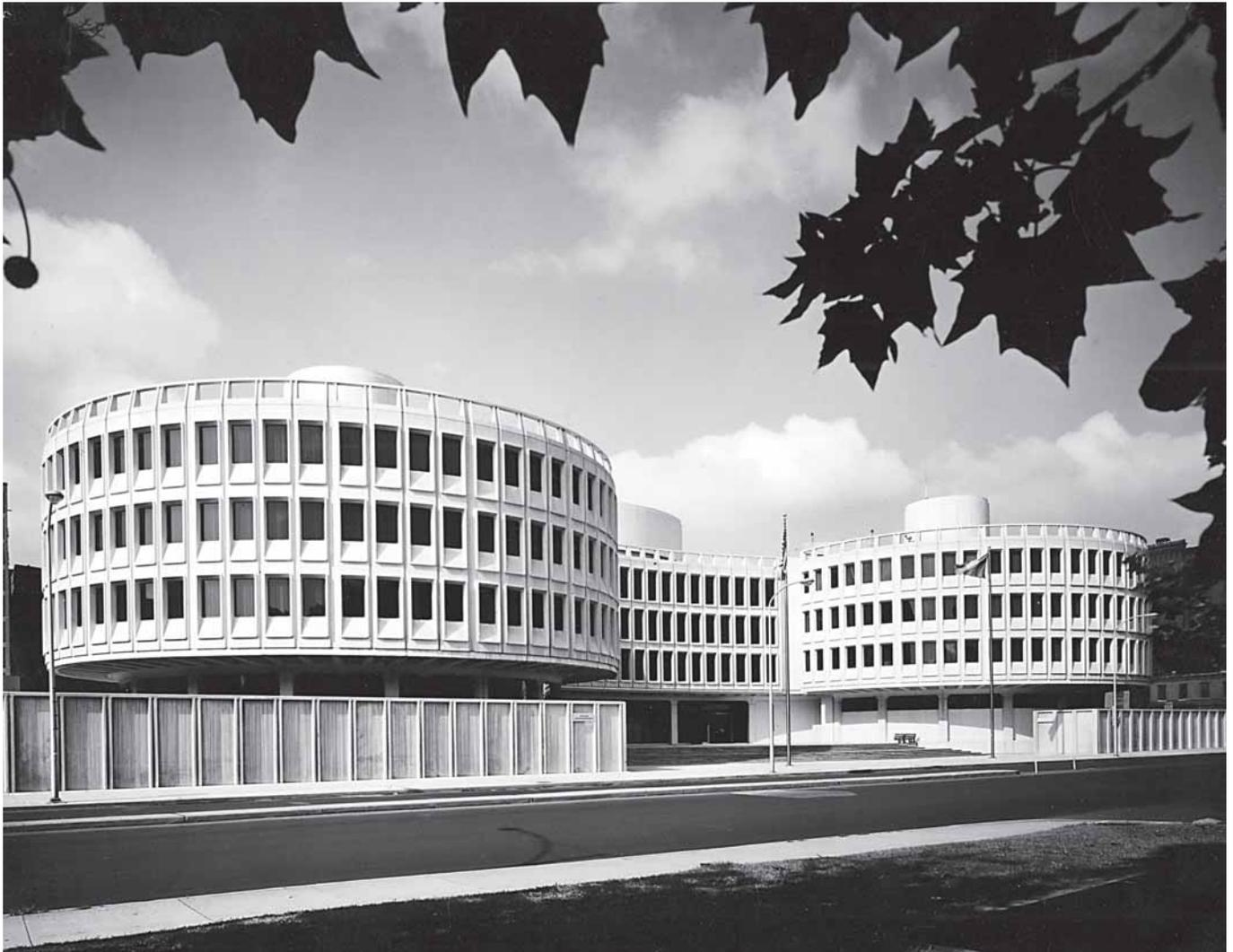
The only cast-in-place concrete above the foundation in the Philadelphia Police Administration Building was the elevator-staircase core. The rest of the superstructure was precast and prestressed.
