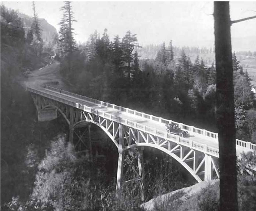
Laturrelle Falls Bridge on the Columbia River Highway, built for the Oregon State Highway Commission in 1914, was one of the first concrete bridges in that state. The bridge was considered one of the lightest concrete structures for the load it carried until the advent of prestressing. Engineer-Architect: K. P. Billner. Builder: Harris Construction Co. *ACI archives. Photo courtesy of K. P. Billner.*
