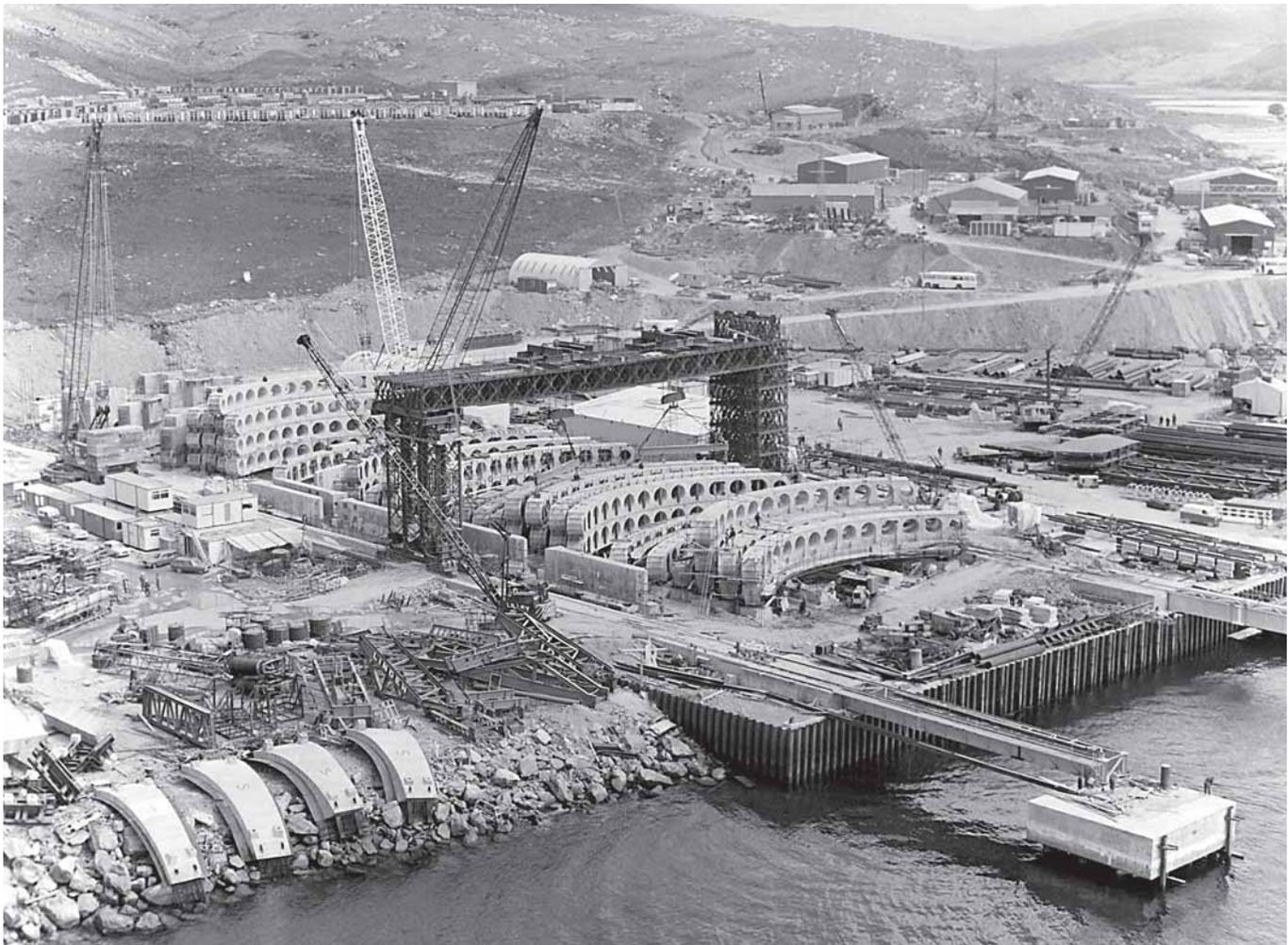
The Ninian Central Platform, a concrete gravity base for drilling and oil production, became the largest floating object built by man when it was towed to location in the North Sea in 1978. The Jarlan-type breakwater wall that crowned the concrete structure was built by assembling rows of quadrant-shaped precast units in a mammoth assembly yard.
