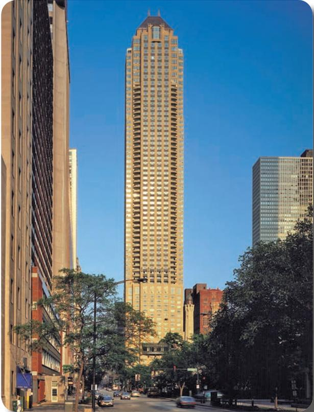
**S**oaring 67 stories above Chicago's Miracle Mile, Park Tower is one of the world's tallest buildings to be clad with architectural precast concrete panels.
