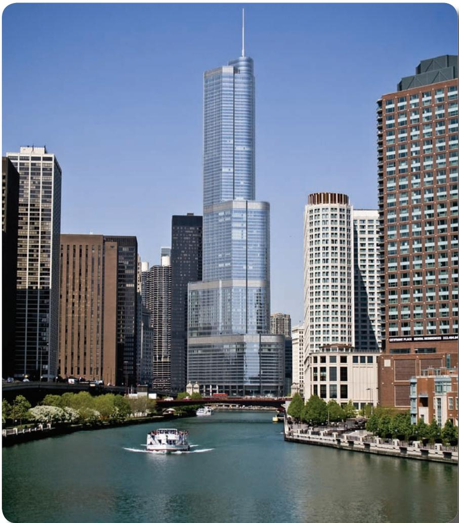
**A**t 1389 ft tall, the 92-story Trump International Hotel and Tower, designed by Skidmore, Owings & Merrill LLP, is the tallest concrete building in the United States. Cutting-edge concrete technologies are used in this reinforced concrete core-wall and outrigger structure, with high-performance mixture designs that include compressive strengths up to 16,000 psi, specified minimum elastic modulus, and self-consolidating concrete.
