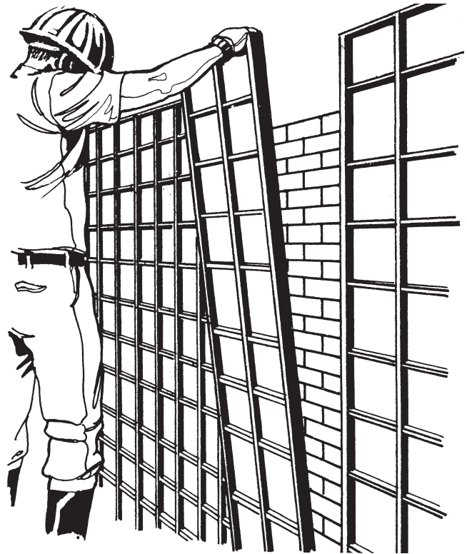
Fig. 5.6 — Cast aluminum forms with a patterned face produce a brick texture in the concrete wall.
