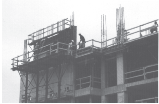
Fig. 5.14 — Jump forms in use. (Photo courtesy of PERI Formwork Systems, Inc.)
