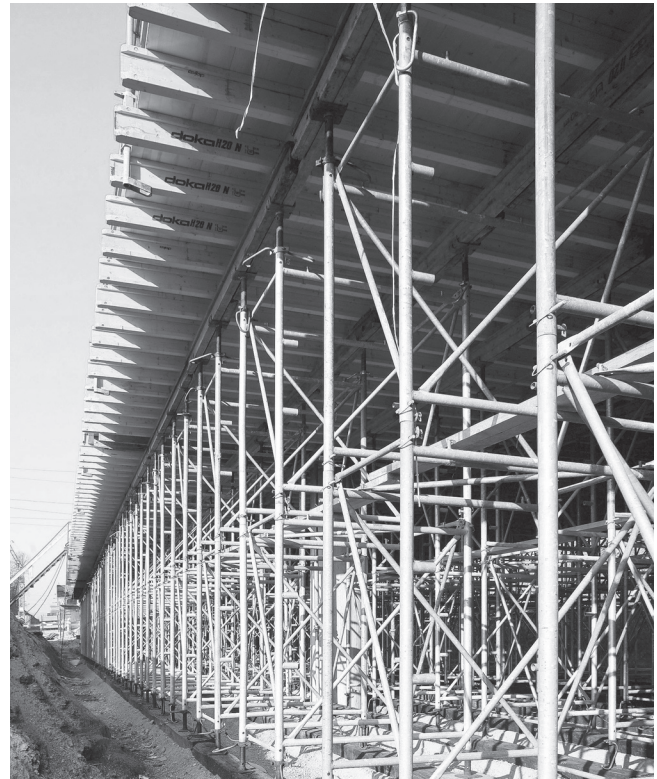
Fig. 5.24 — Tubular welded frame shoring. (Photo courtesy of Doka Group.)
