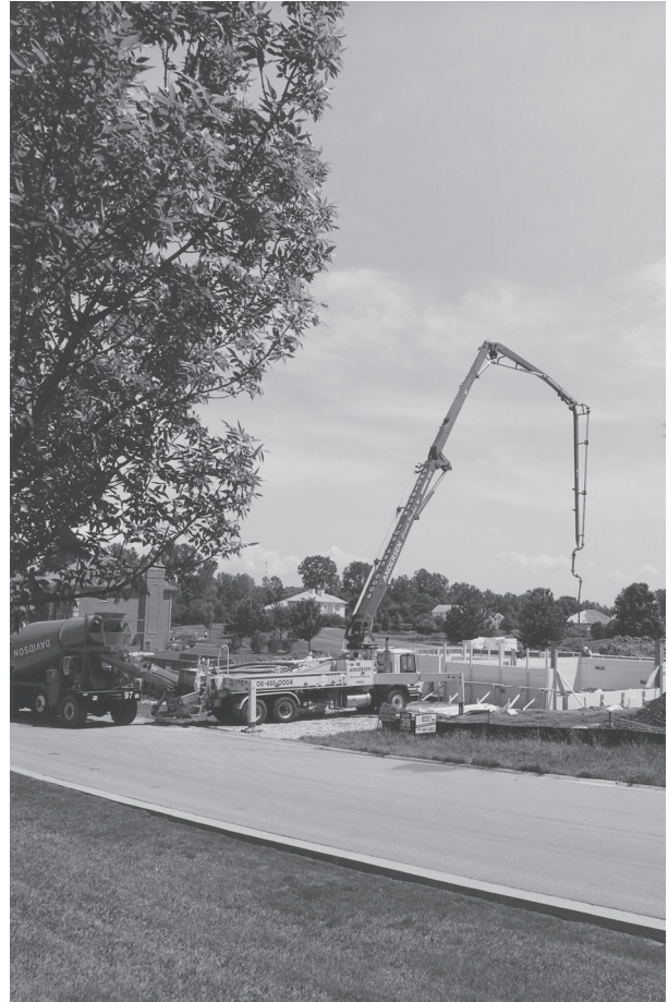
Fig. 5.12—Insulating concrete forms (ICFs) are assembled and then filled with concrete. (Photo courtesy of Schwing America Inc.)
