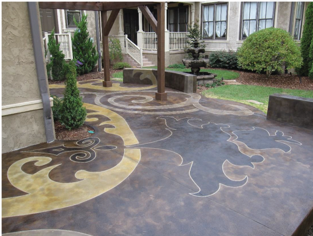
Fig. 1.2a—Cast-in-place decorative concrete combining treatments during and after placement to achieve aesthetic effects (courtesy of Concrete Mystique Engraving).
