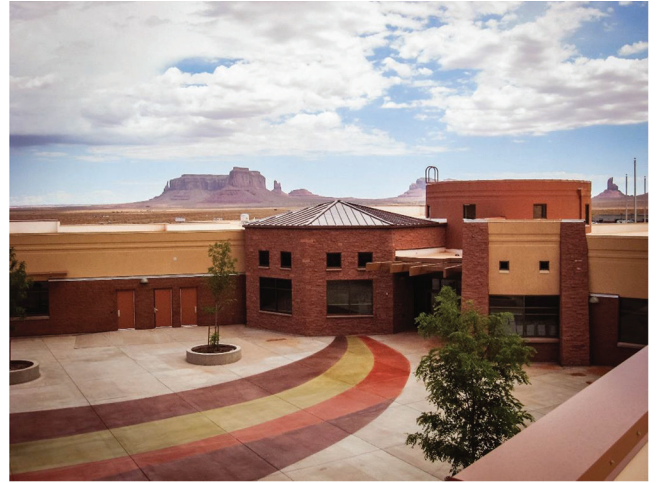
Fig. 1.2b—Decorative concrete applications such as post-placement colorants can complement or enhance the overall aesthetics of a project (courtesy of PROSOCO).
