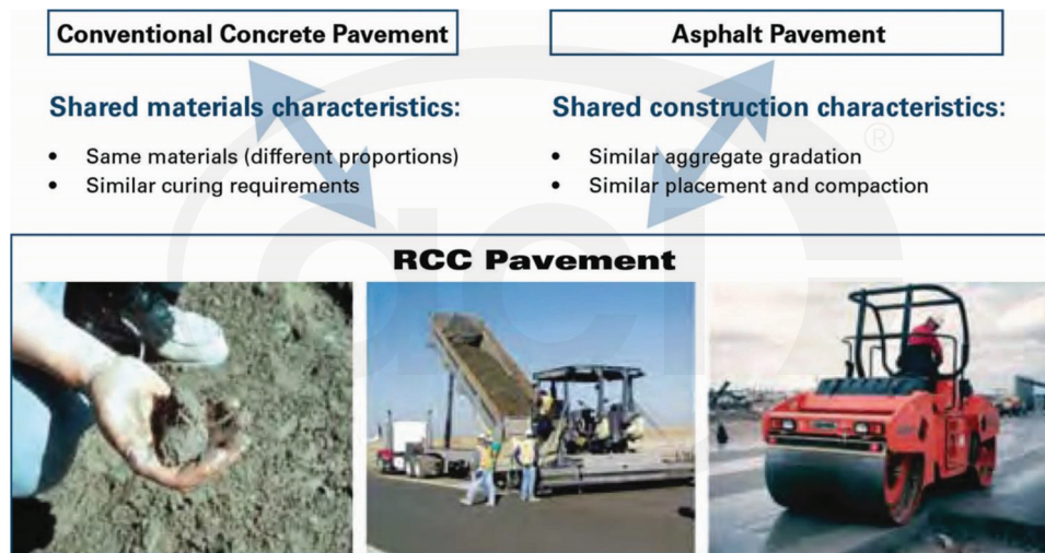
Fig. 3.2a—RCC combines aspects of conventional concrete and hot-mix asphalt paving materials and construction practices (Harrington et al. 2010).
