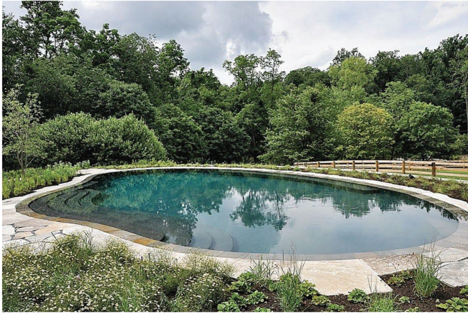
Fig. 1.1—Curved pool with close-tolerance high water level. No straight or flat sections.
