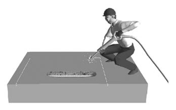
Fig. 4—Initial concrete removal within the sawcut area, using a 15- or 30-lb jackhammer. Use 15-lb jackhammer for final removal.
