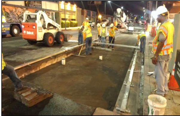
Grading Bedding Material
