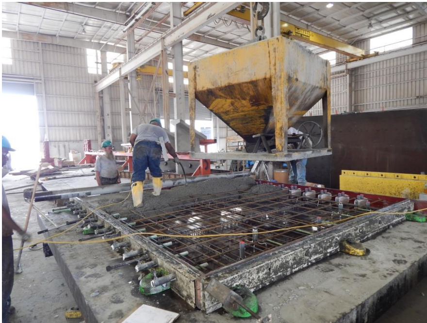
Spud vibrator used for consolidation.
