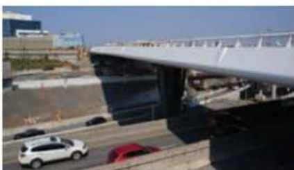
View of the Saint-Jacques Bridge before installation of the main pillar
