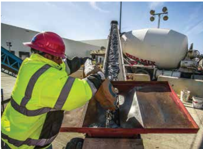
Before each concrete truck entered the building, steel fibers were added at a dosage of 23 lb/yd 3 (13.6 kg/m 3 ) (photo courtesy of Jon Humphrey)
