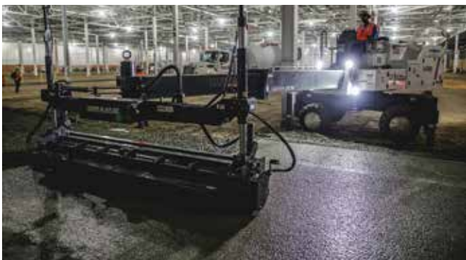
Four laser screeds were used during the placement, helping to provide a slab surface that was within 3/16 in. (5 mm) of plane over the huge floor area (photo courtesy of Jon Humphrey)
