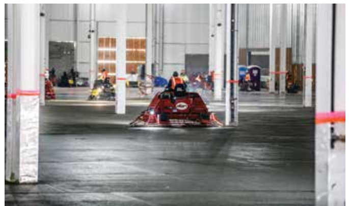
The operators of 38 ride-on trowels made sure that the finished floor had high FF/FL numbers—achieved values were 56/42 (photo courtesy of Jon Humphrey)
