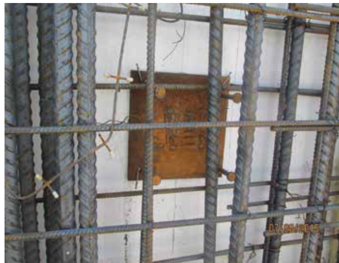
Fig. 6: Embed plates require small diameter holes for installation on wall form (photo courtesy of Ceko Concrete Construction)
