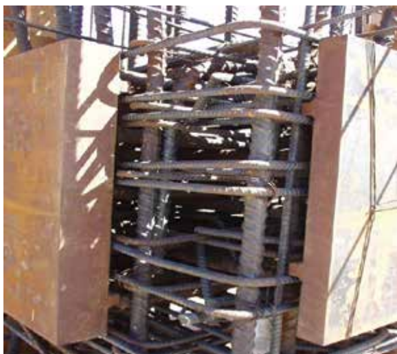
Fig. 3: Reinforcing bars must clear embed plates and studs by the clearance provided in Section 2.3.1 of ACI 117, and the SER must provide details showing how the clearance is to be maintained. This is particularly critical when the embeds have very thick plates (photo courtesy of Bruce Suprenant)
