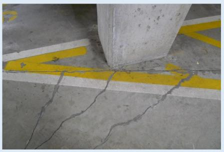
A four-story, cast-in-place concrete parking garage, suffered excessive slab cracking soon after construction.
