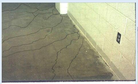
A three-story, cast-in-place concrete educational building, suffered excessive slab deflections and cracking due to premature removal of shores and reshores.
