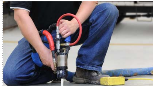
Resin Injection Packer
