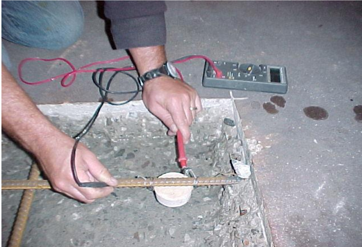
Testing anode connection to reinforcing steel.
