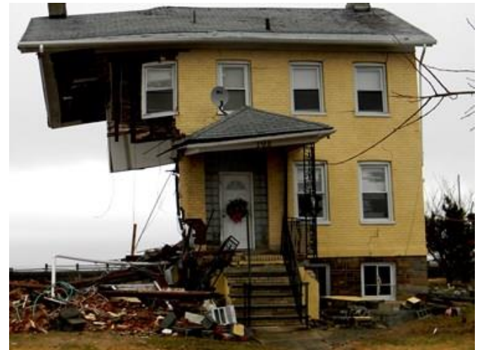
Another home, just three lots down, looked like this following the super storm..
