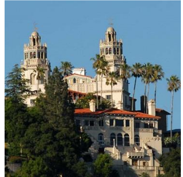
Hearst Castle: Reinforced Concrete Built from 1919-1947; Suffered no damage in 2003 from four earthquakes .
