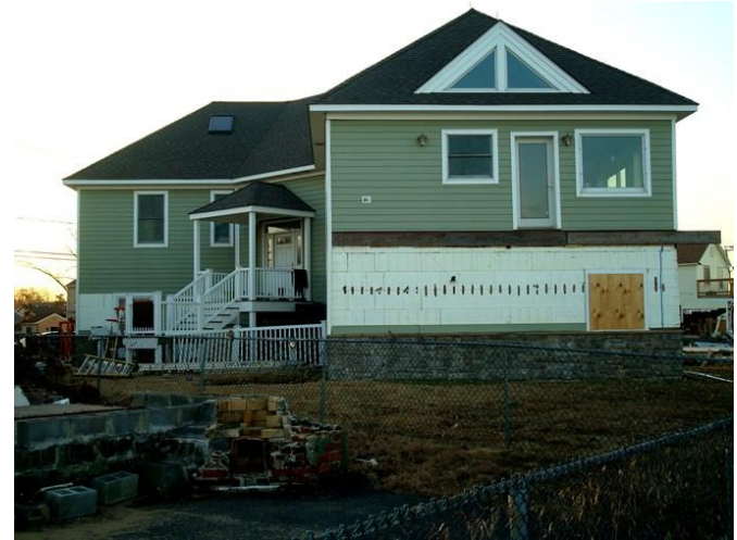
After Hurricane Sandy, the ICF home was structurally intact, with only a section of exterior siding missing.
