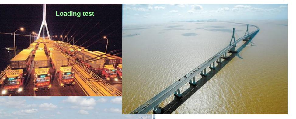
**Design life: 100 years** Quad blend (PC/GGBS/FA/SF) Built in less than 3 years. Speed limit 50mph...
