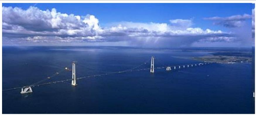
Length of free span: 1,624m Height of pylons: 254m Main channel clearance: 65m Concrete volume: 380,000m<sup>3</sup>
