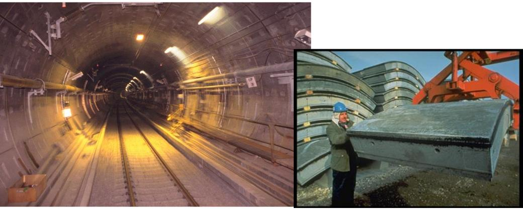
Two parallel 8,500m sub sea tunnels = 62,000 precast concrete lining elements
