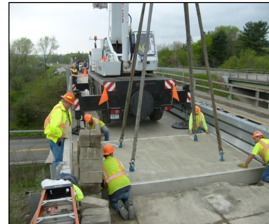
Placing panels In One Lane
