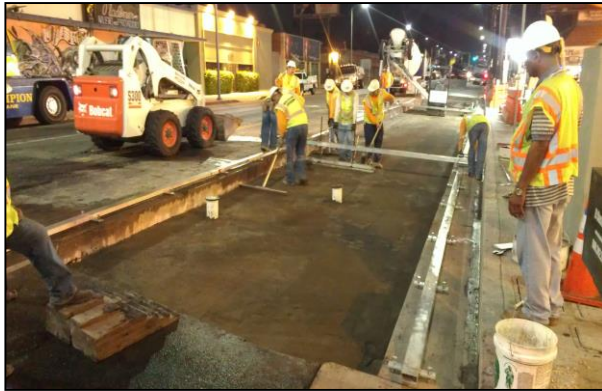
Grading Bedding Material
