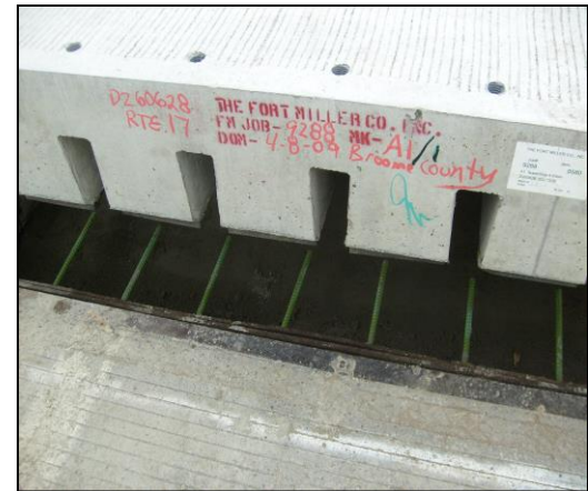
Placing panel Over Anchor Rods
