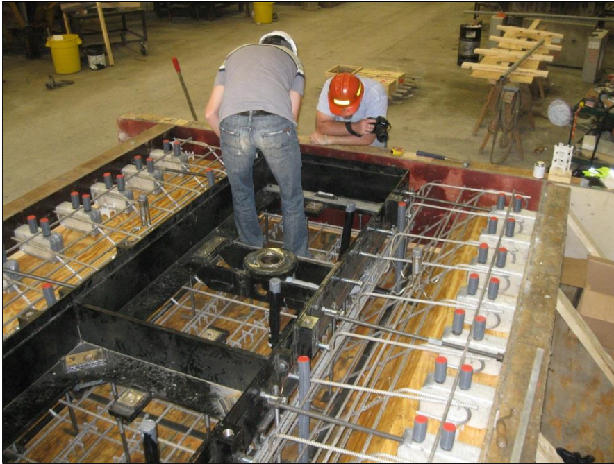
Fabrication Stainless Steel Reinforcing and Dowels
