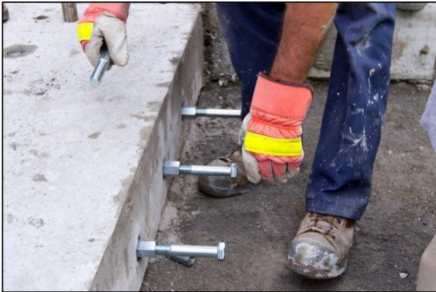
Restoring Tie Bars
