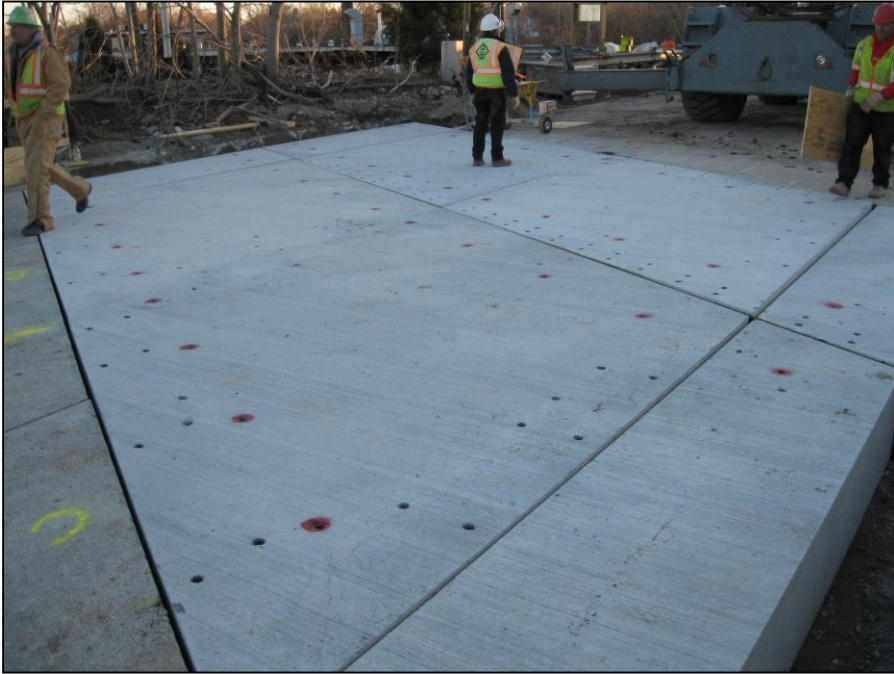
Skewed and Warped Panels
