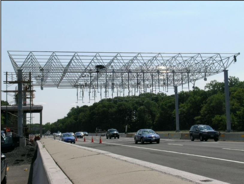
Open Road Tolling
