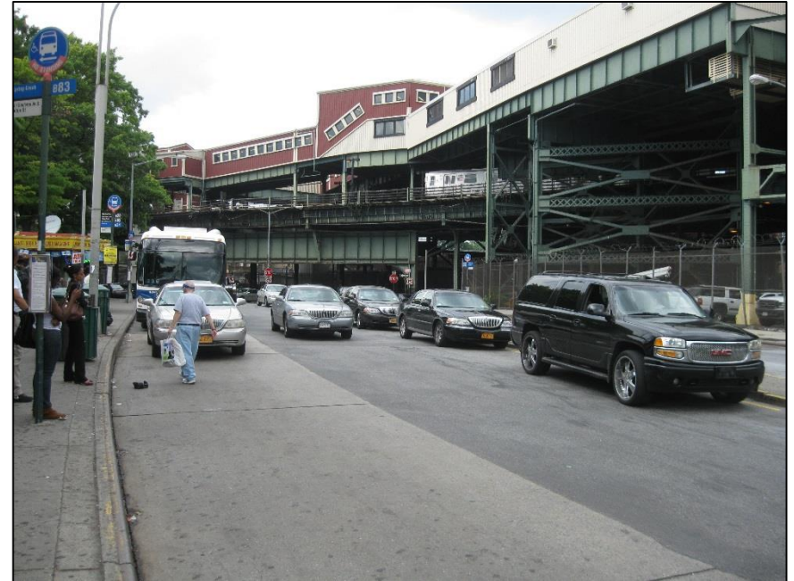
Looking South (Bus Pad on Left)
