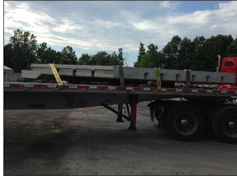
Haunched & Notched on Top for Bridge Joint
