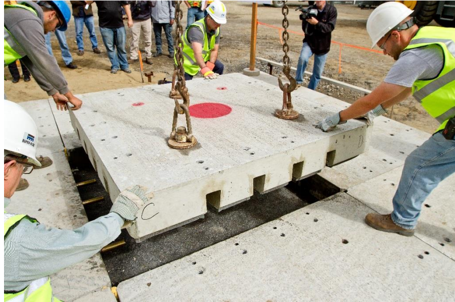
Replacing Cleaned-Up Panels
