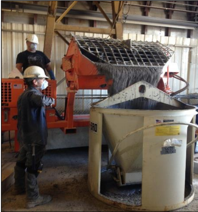
Mixing Polymer Concrete
