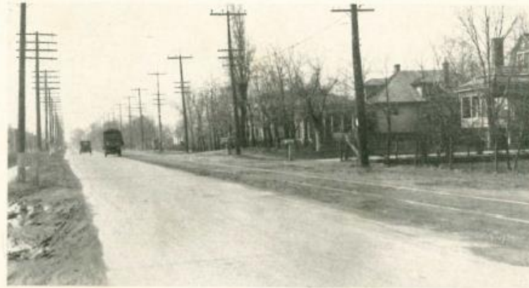
South Seventh Street Road, Terre Haute, Ind., showing condition of concrete resurfacing after 8 years' service.
