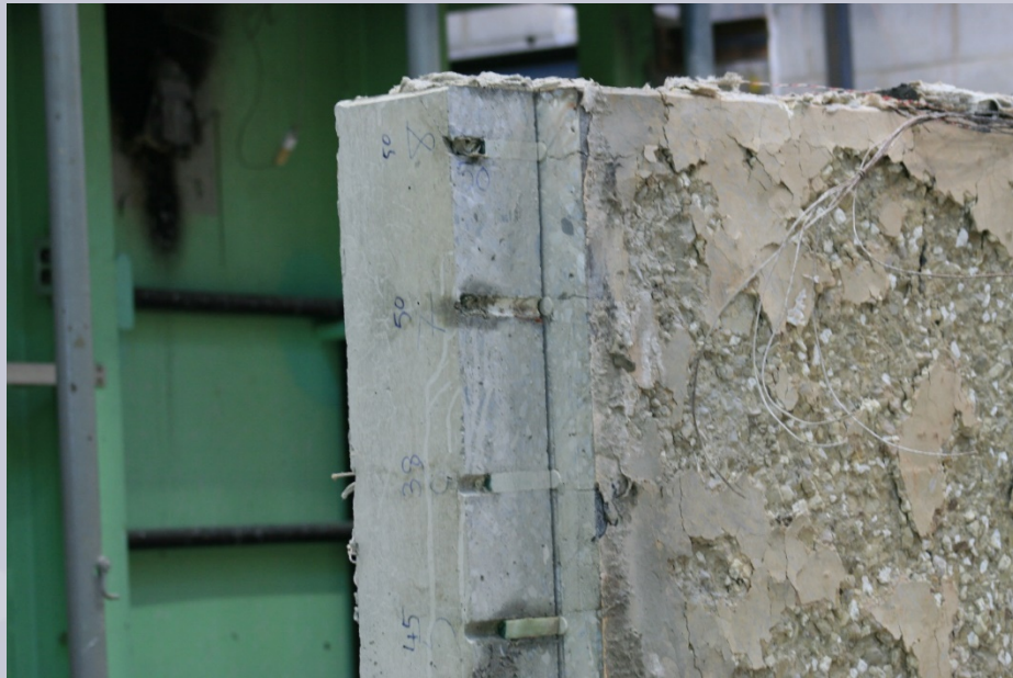
All FRP bars were pulled out at one end of Slab-B.
