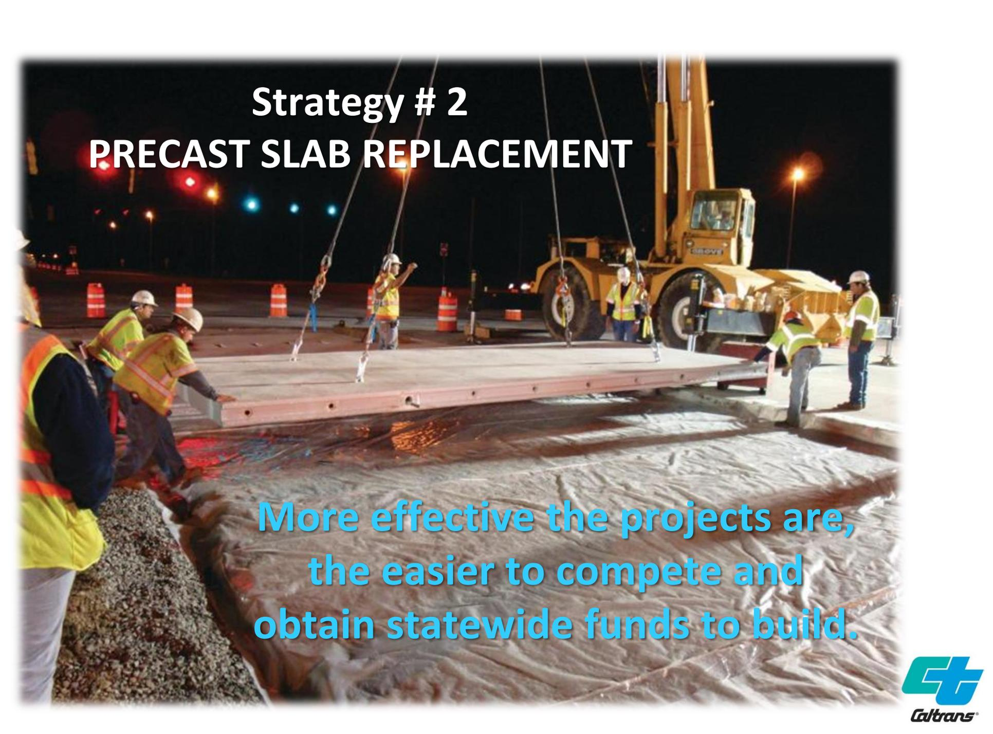
A photograph of a construction site at night. A large yellow crane is lifting a long, rectangular precast concrete slab into a trench. Several workers in high-visibility vests and hard hats are positioned around the slab, some holding ropes attached to the crane. The ground is covered with a white plastic tarp. In the background, there are orange traffic barrels and streetlights.
