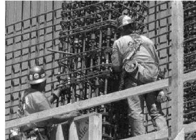
Detailing columns with mechanical couplers can help reduce congestion and improve constructability (photo courtesy of Tipping Structural Engineers)
