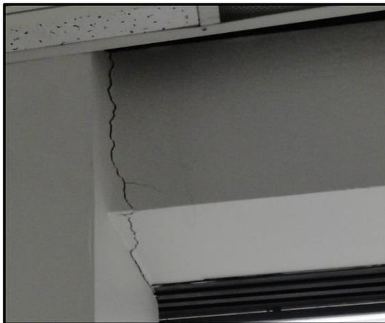
Single crack in beams (with min. reo) is an indicator of low rotation demands
