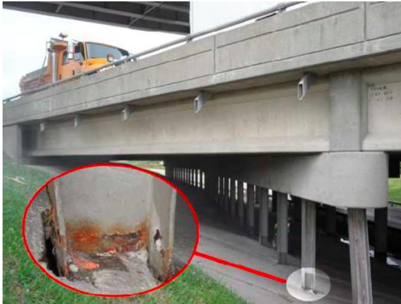
One of the 49 Corrosion-damaged piles in I-70/I-270 interchange (St. Louis, MO) that were repaired with this technique
