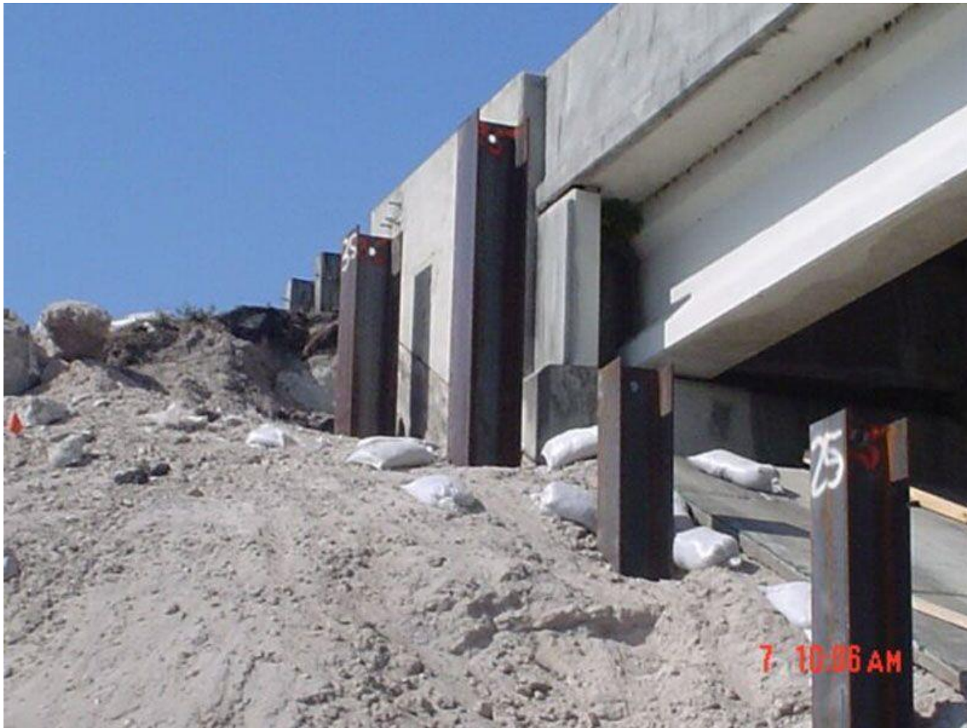
Steel HP piles used in conjunction with sheet piles
