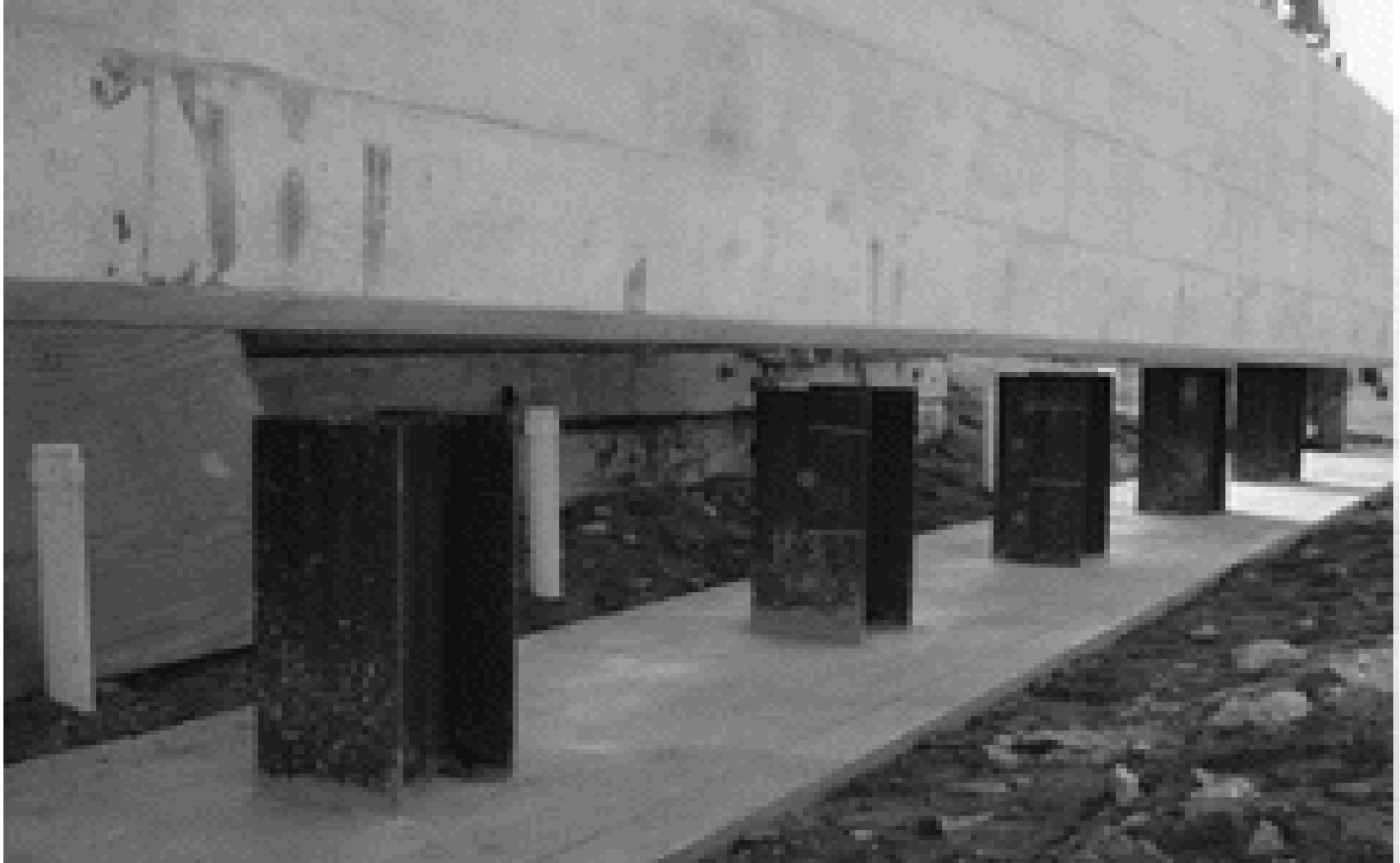
Steel HP piles used for abutment foundations
