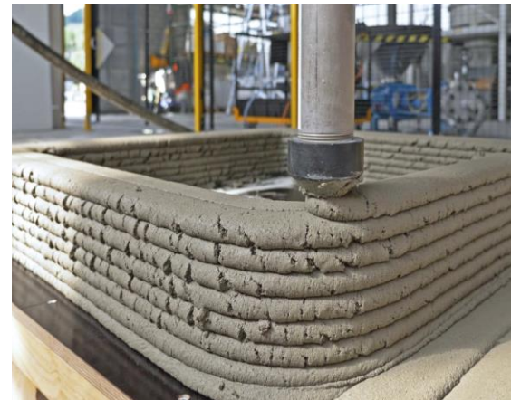
Plastic shrinkage cracking
