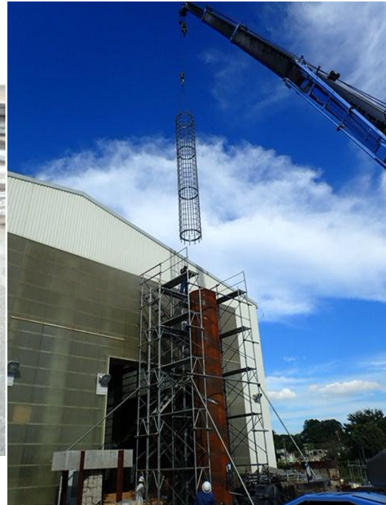
Placing reinforcement cage in a steel tube
