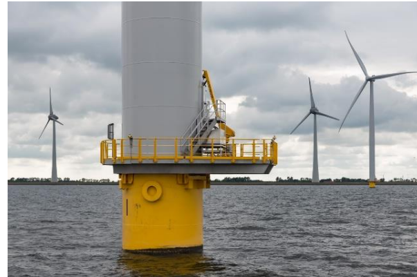
Offshore wind turbine foundations
