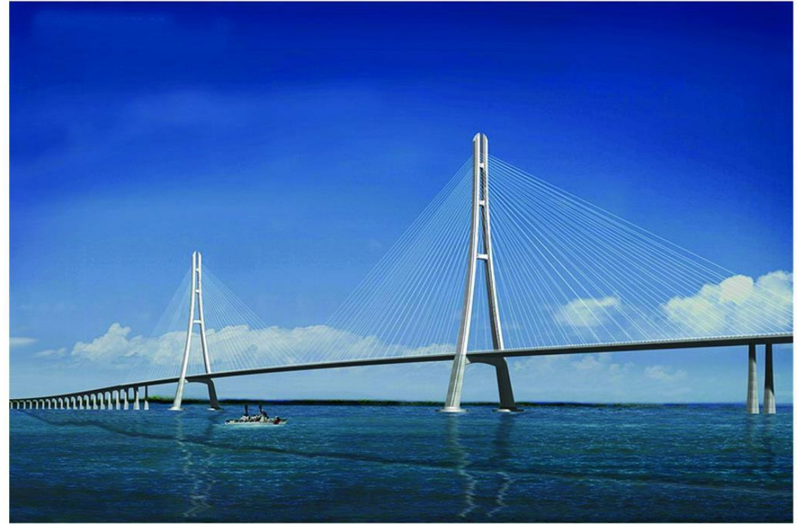
(b) The Nanjing Dashengguan Yangtze River Bridge in China
