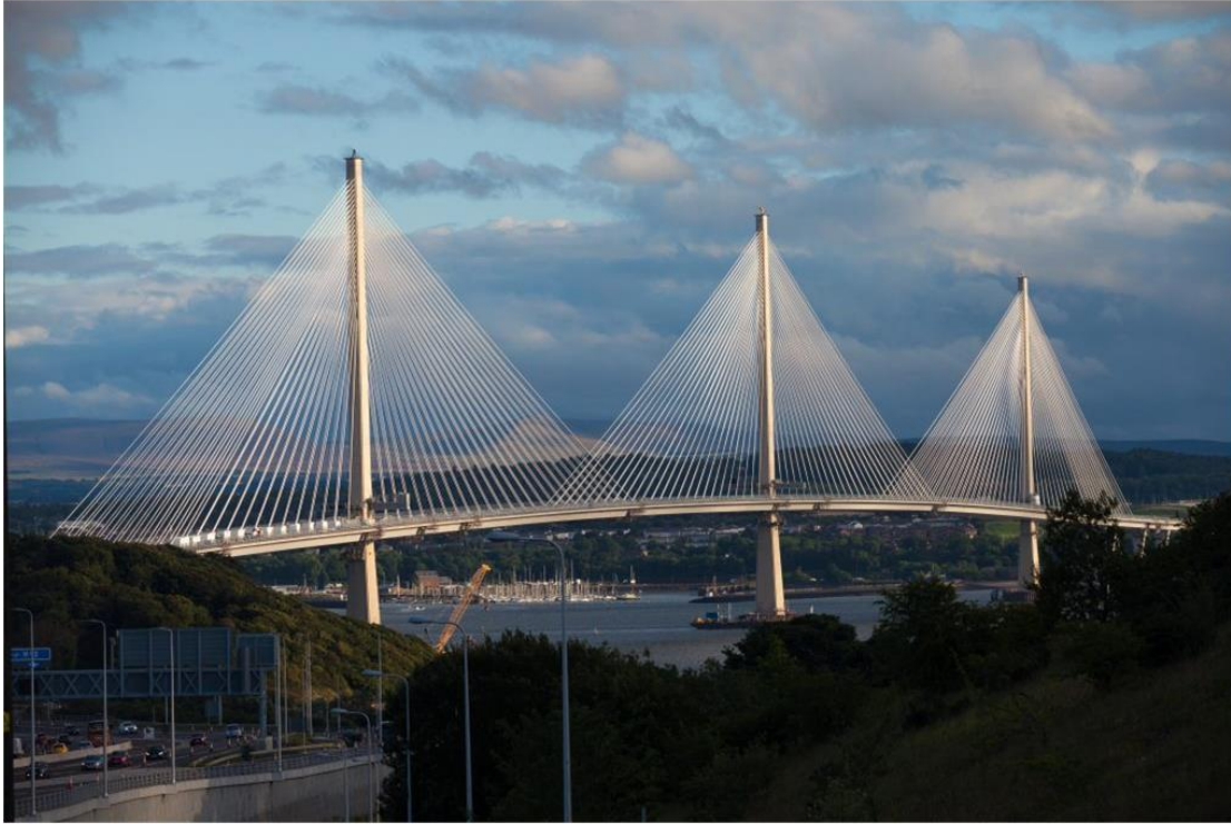
(a) The Queensferry Crossing in the UK
