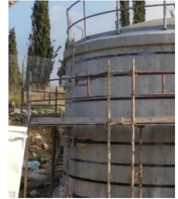
Reinforcement of silos and water tank (round shape)
