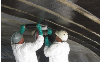
EXTERNALLY BONDED FRP OR STEEL
