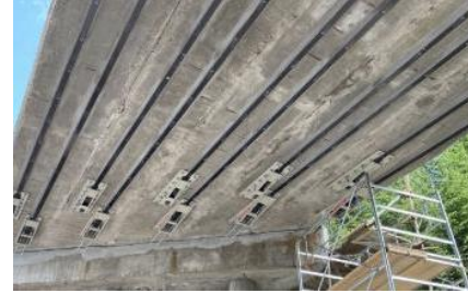
EXTERNAL POST- TENSIONING
