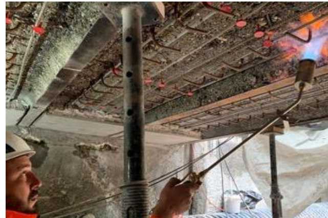
Heat activated NSM Fe-based shape memory alloy rods 1-2
