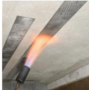
Heat activated NSM Fe-based shape memory alloy plates
