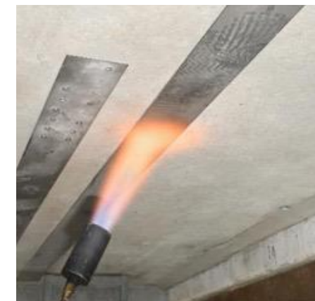
Heat activated Fe-based shape memory alloy plates 3
