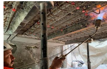
Heat activated NSM Fe-based shape memory alloy rods
