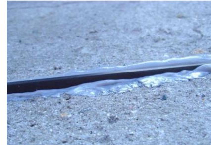
NSM FRP rods and strips
