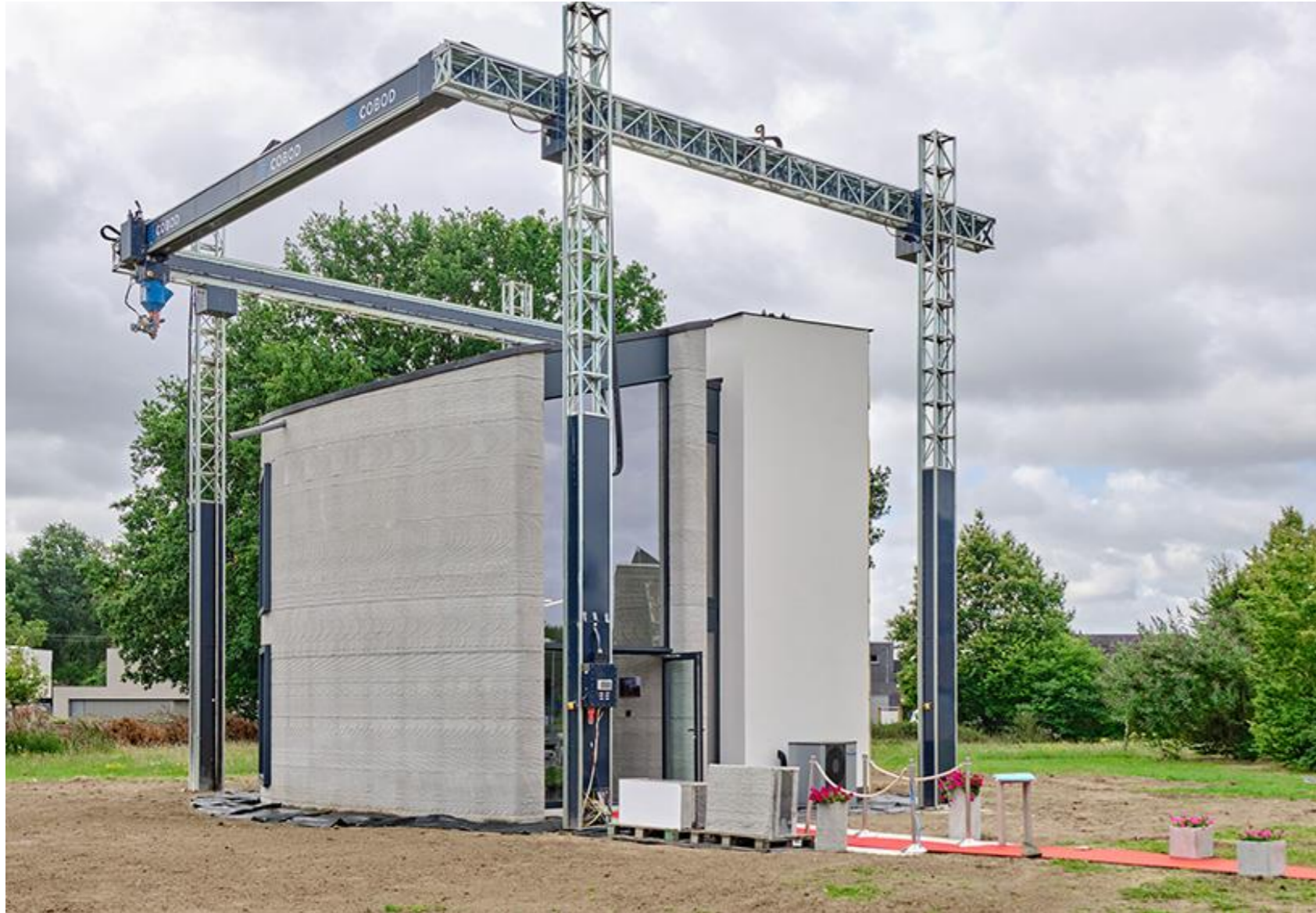
(First 3DCP house in Belgium)
