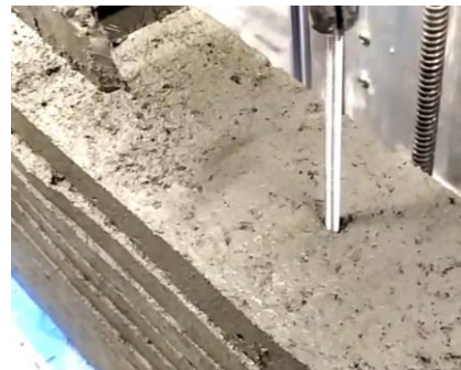
Reinforcement integration process
