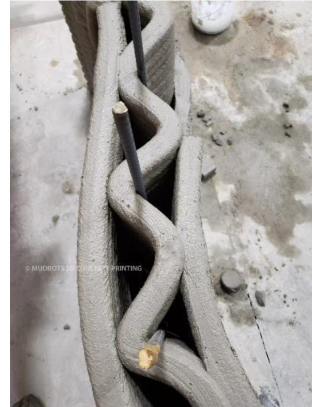
Hybrid Construction (printing formwork, reinforcement placement & casting)
