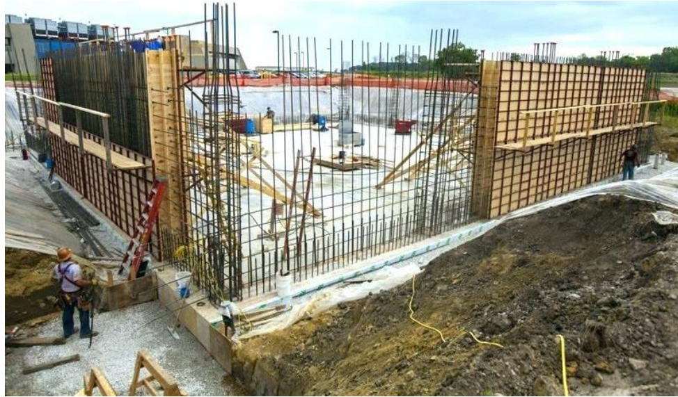
Conventional Construction (forming, reinforcement placement & casting)
