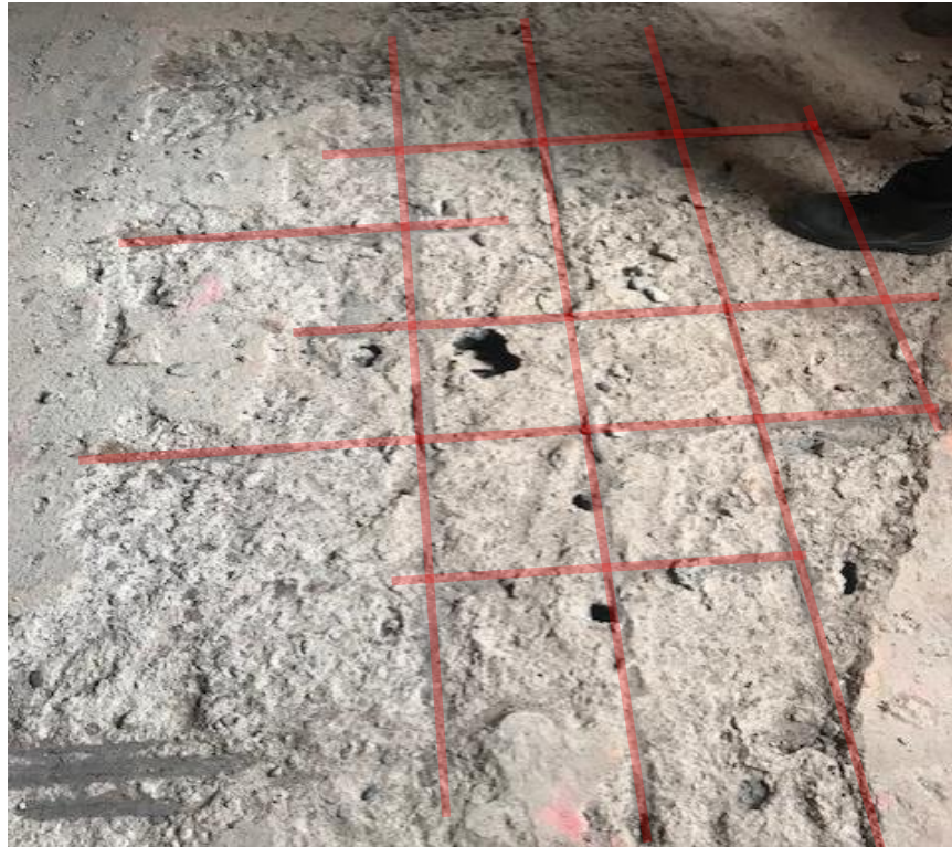
(a) Before strengthening
