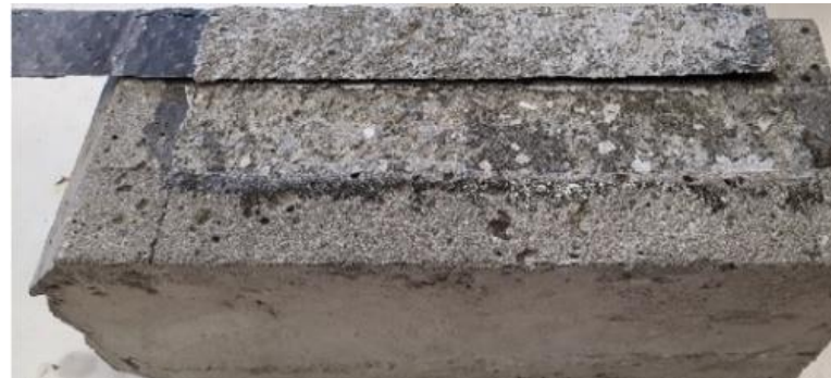
Mixed failure in concrete and adhesive/concrete interface (200 cycles)
