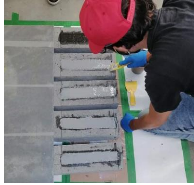
3. Applying the adhesive layer (epoxy paste).
