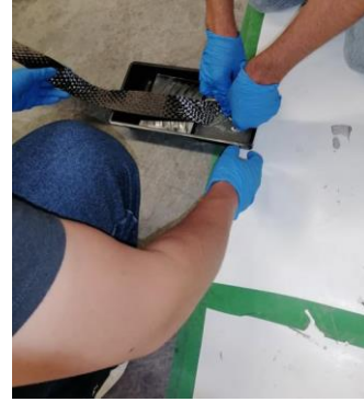
4. Impregnation of the carbon fiber fabric strip with epoxy resin.
