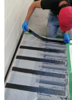
5. Installation of CFRP strips.
