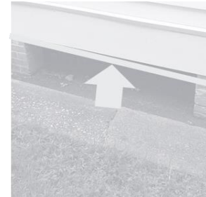
Outdoor, sheltered from rain k = 6.6
