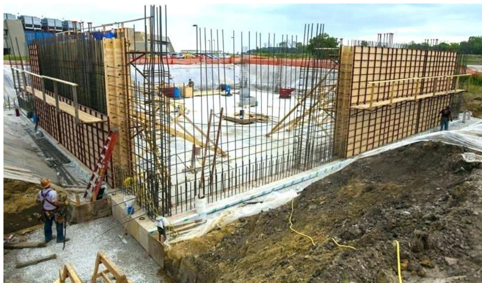
Conventional Construction (forming, reinforcement placement & casting)
