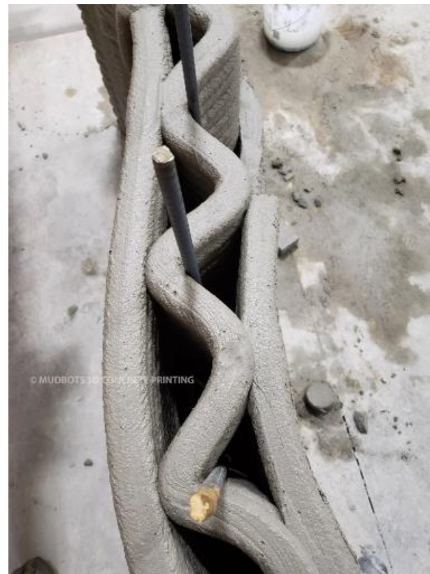
Hybrid Construction (printing formwork, reinforcement placement & casting)
