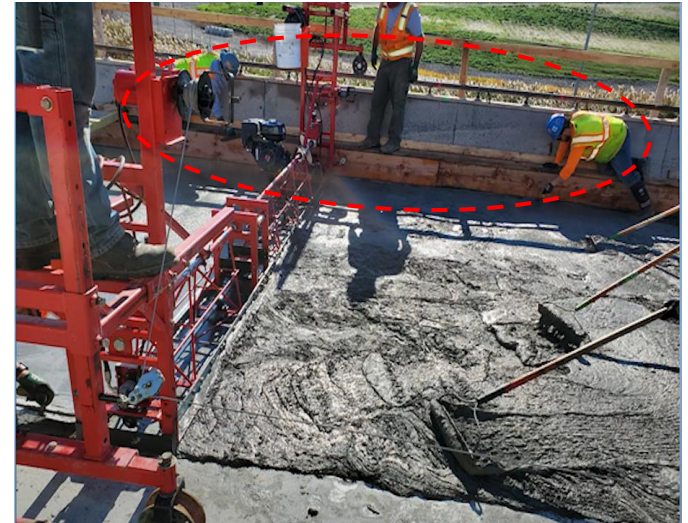
Labors and formworks
