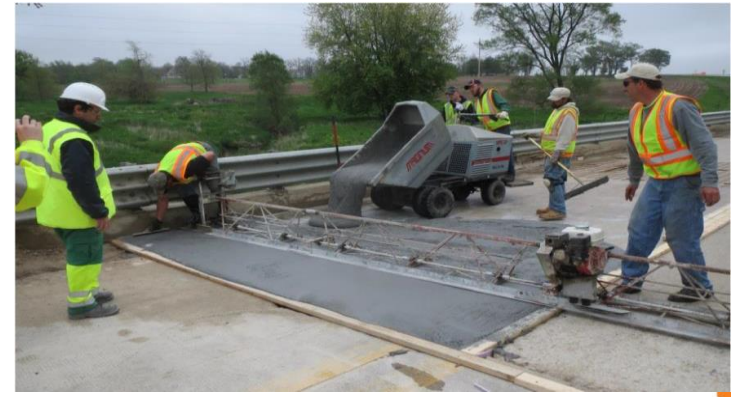
Thin-bonded overlays on bridge decks
