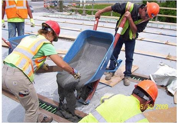
Field-cast bridge deck slab joints
