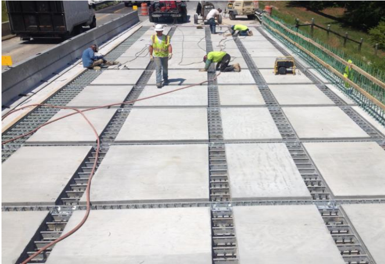
Precast deck panels with transverse and longitudinal joints, photo credit: Georgia DOT)
