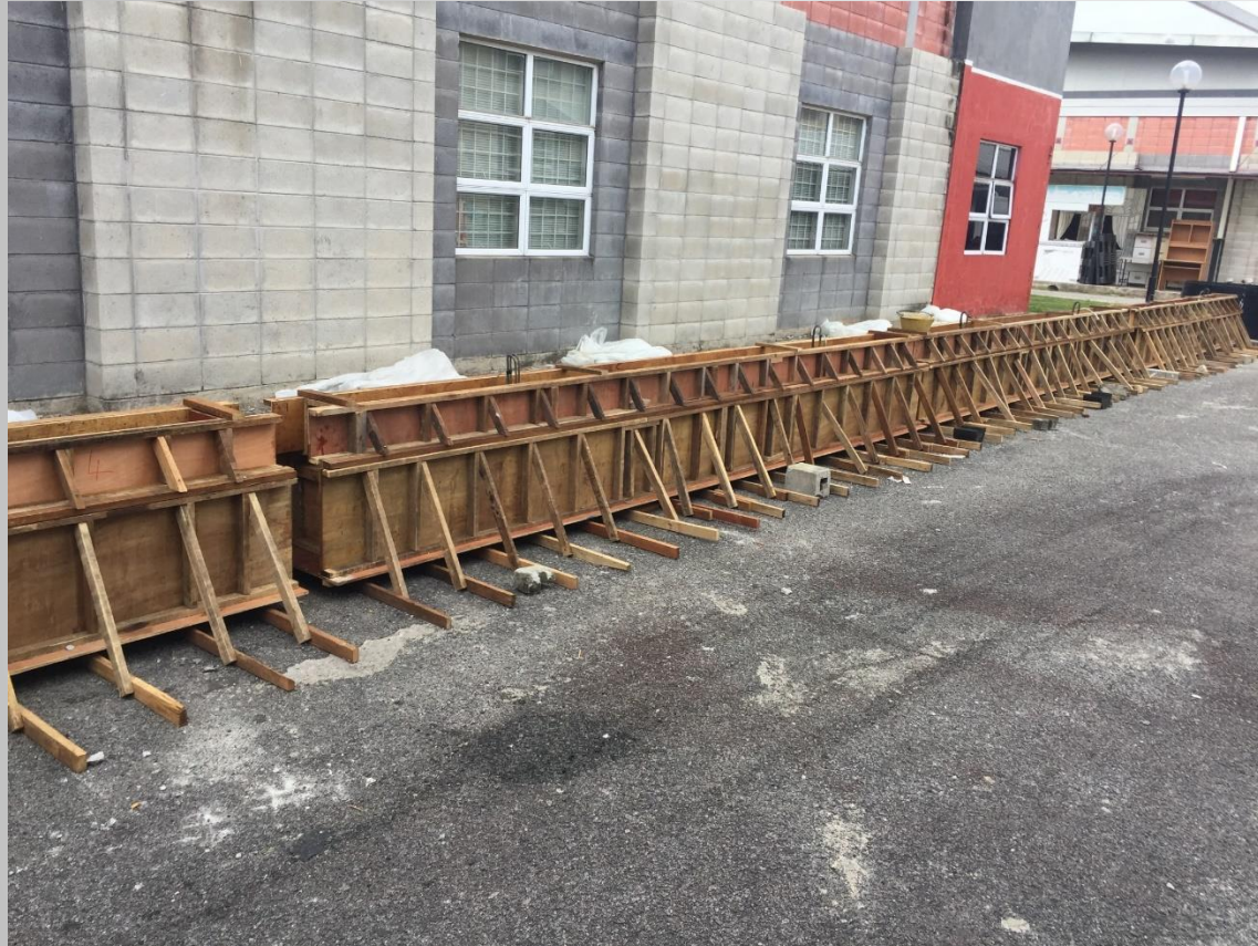
Precast beam ready to concrete
