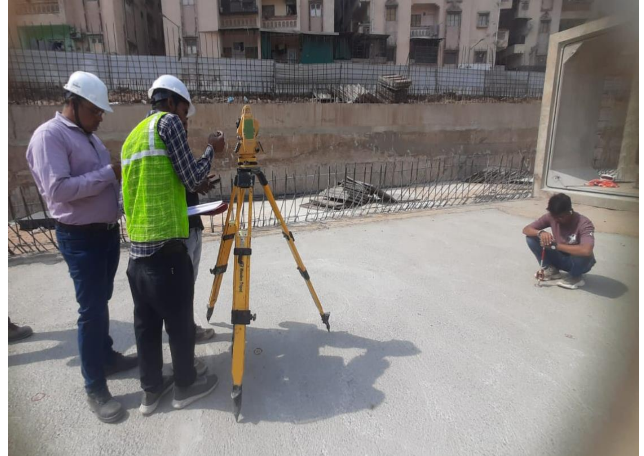
PCC Level Checking and Centerline Survey Demarcation Work
