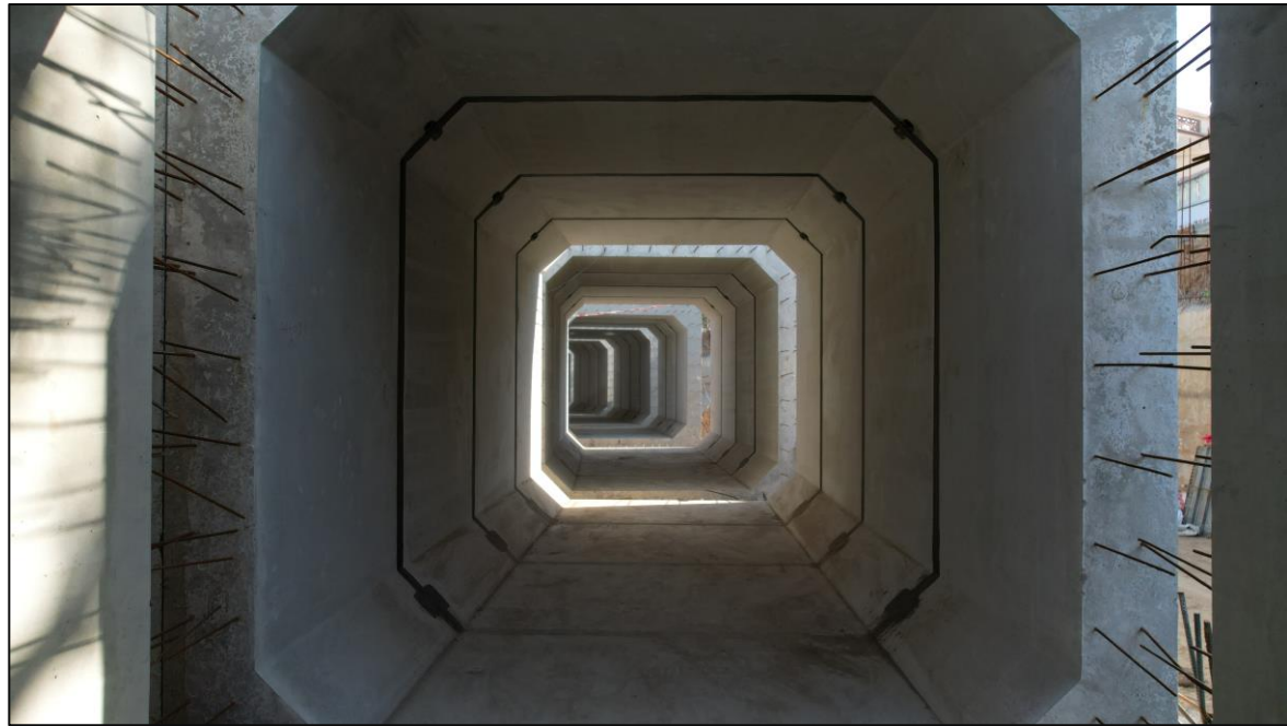
Dowel Box Culvert Joint
