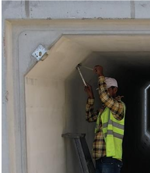
High Tensile Nut-bolt fixing
