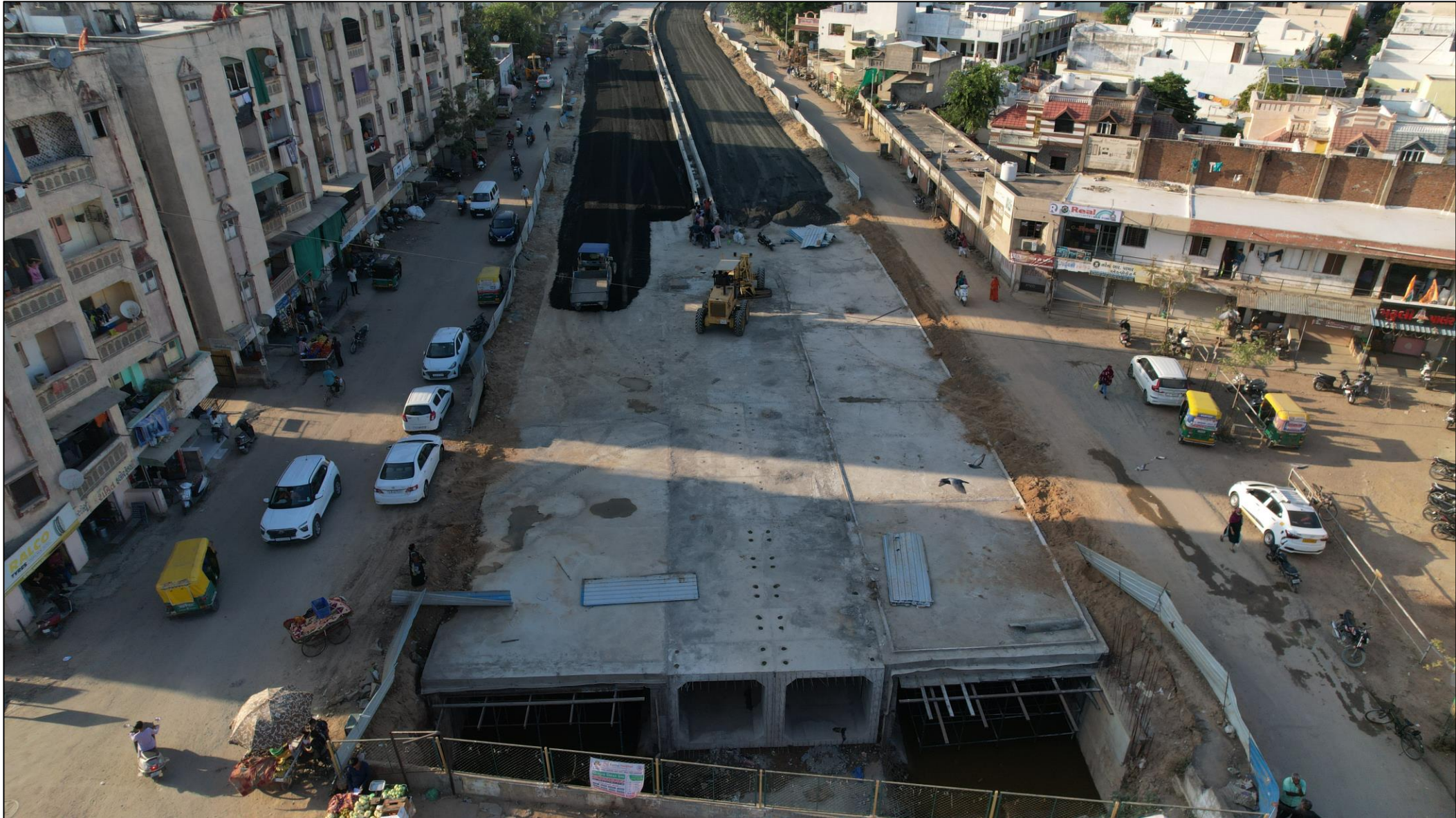
Double Cell Box Culvert Canal
