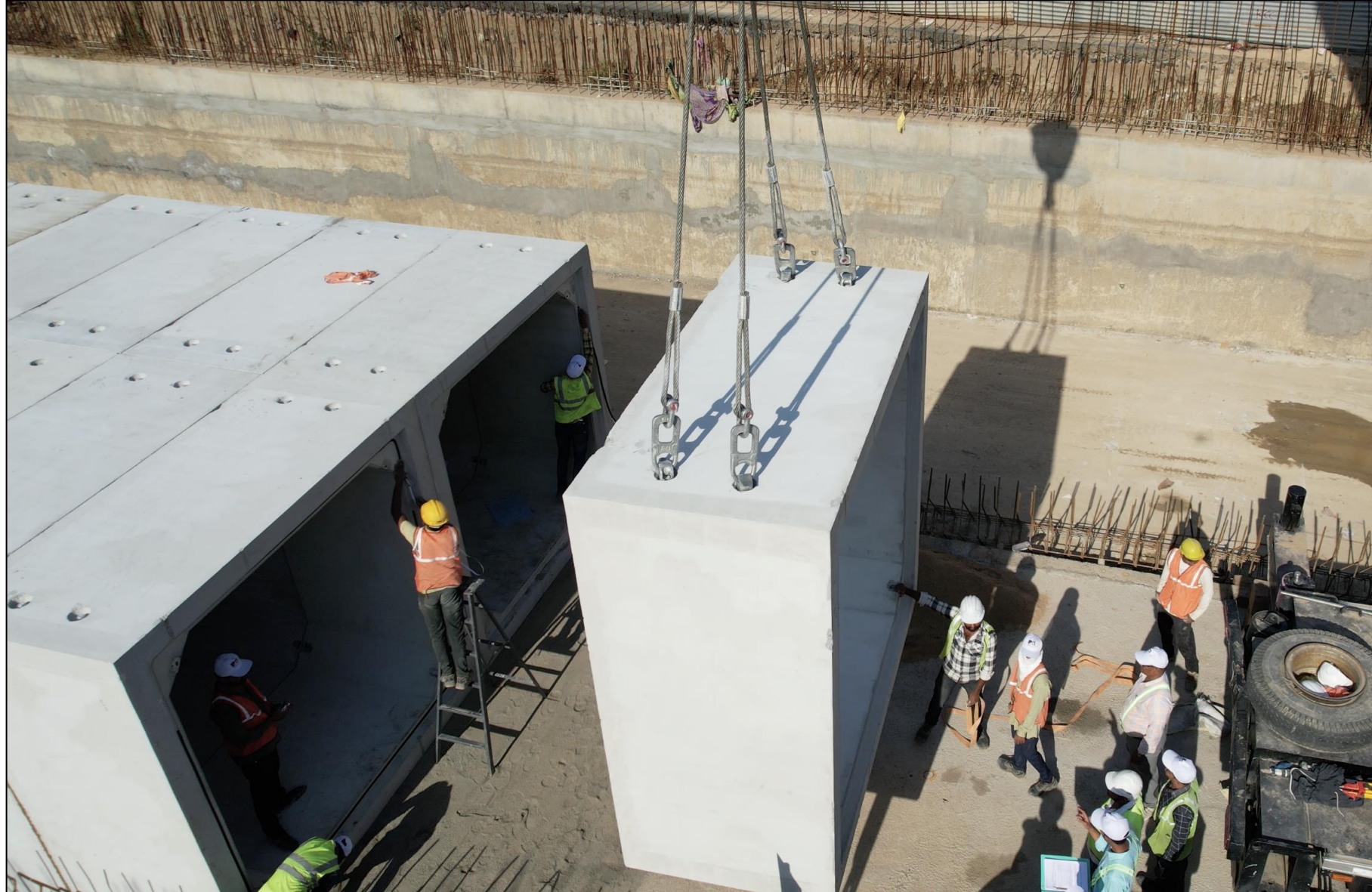
Laying Of Box culvert
