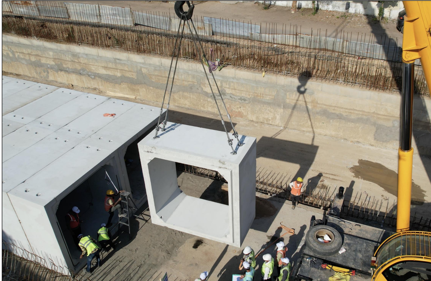
Lifting Of Box culvert
