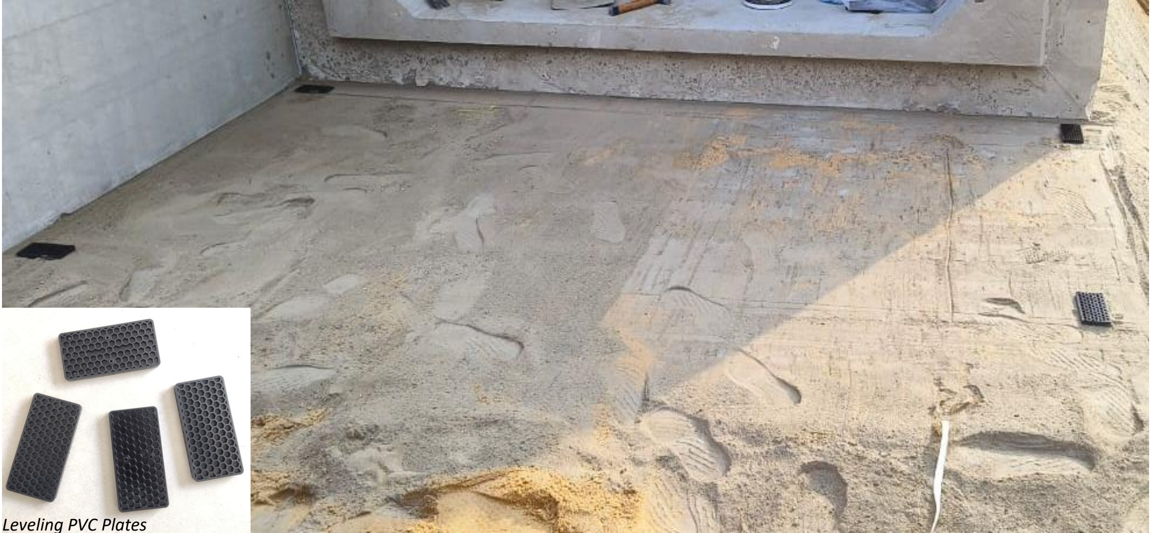
Bed Preparation ( with leveling of Cement Mortar and PVC Plate )
