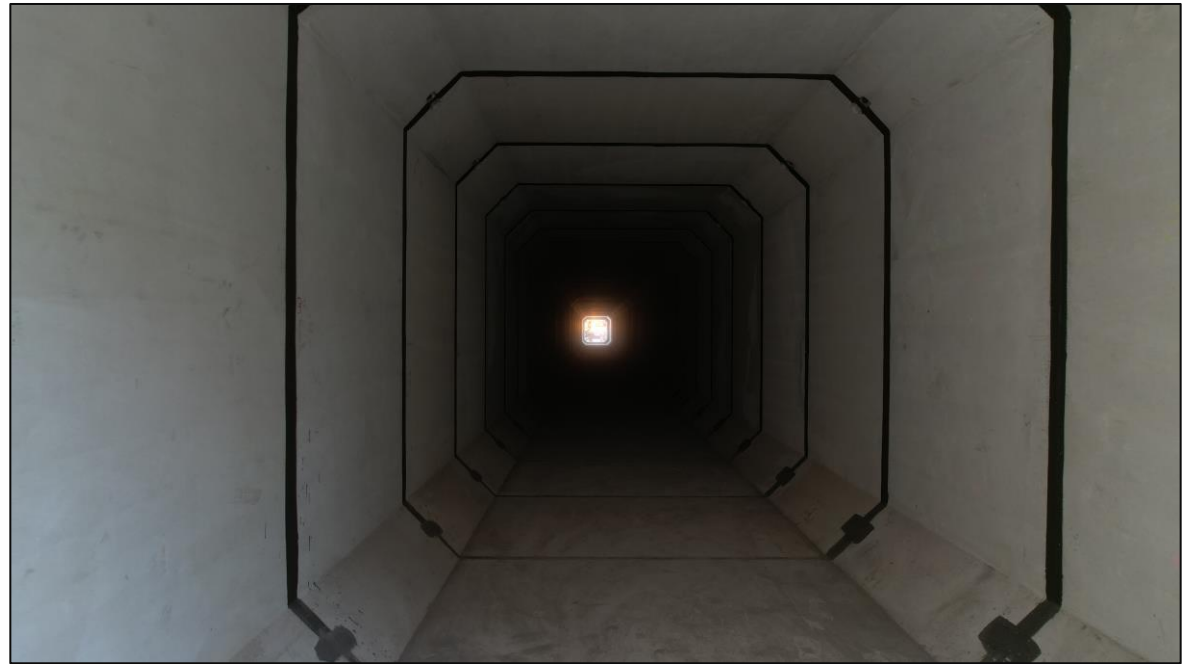
Straight Box Culvert Joints
