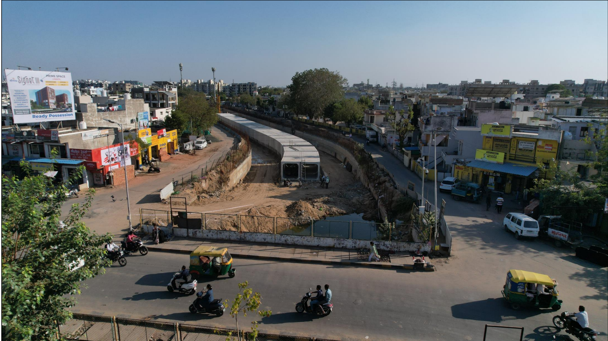
Double Cell Box Culvert Canal
