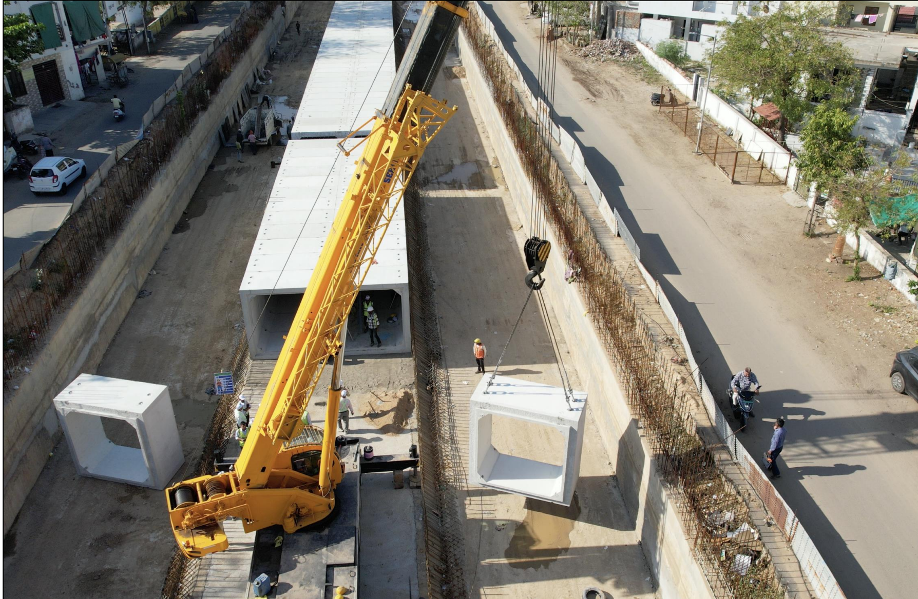
Double Cell Box Culvert Canal
