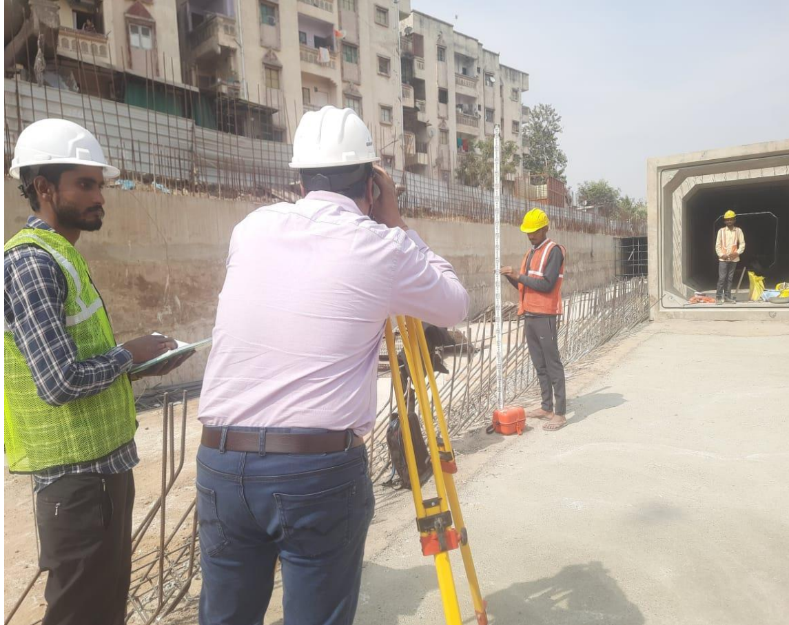
PCC Level Checking and Centerline Survey Demarcation Work
