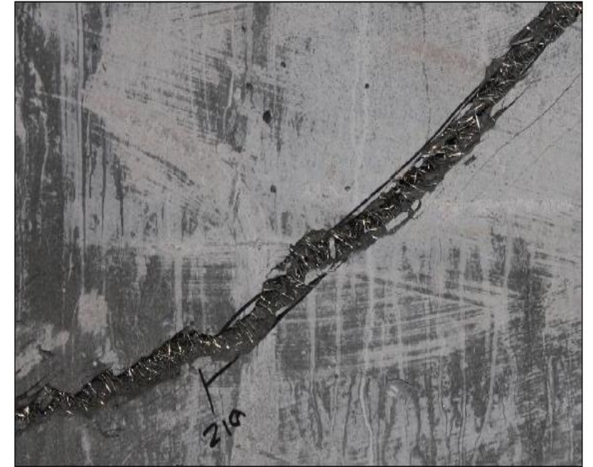
Steel fibers bridge the crack at peak load
