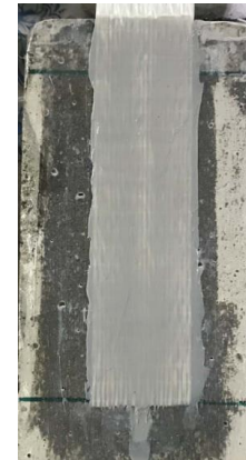
Bonding FRP to concrete
