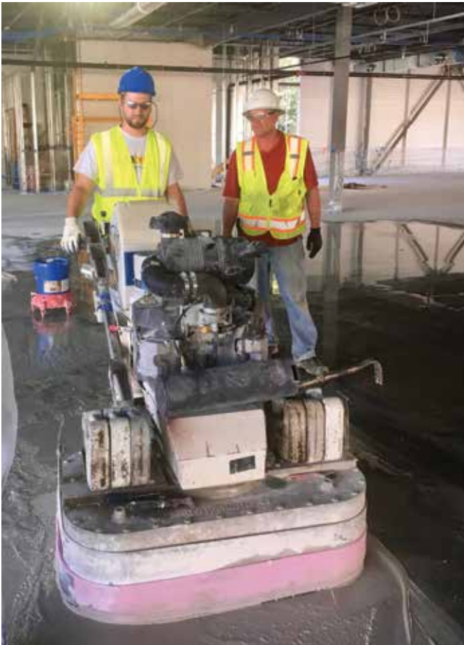
Floor processing begins with wet grinding
