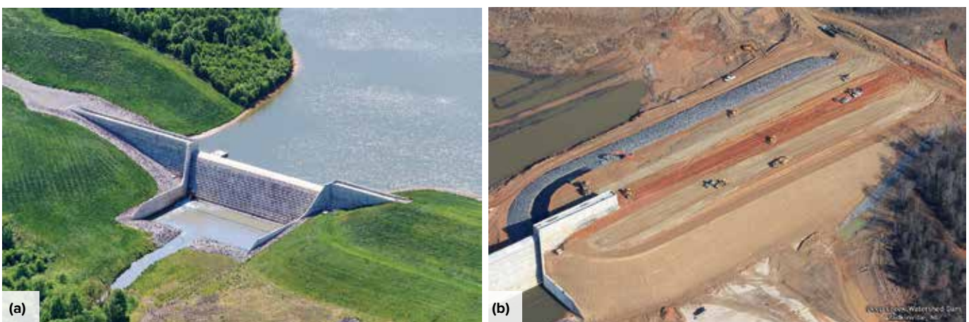
Fig. 1: Deep Creek Dam is a composite dam with an RCC gravity spillway and abutment closure section and an earth embankment section: (a) completed dam (© photo courtesy of Aerial Photo Pros); and (b) construction of the earth embankment section (© photo courtesy of Sky Site Images)
