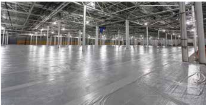
Curing of the finished Mega Slab was accomplished using polyethylene sheeting with a saturated superabsorbent polymer backing. The sheeting was left in place for 7 days (photo courtesy of Jon Humphrey)
