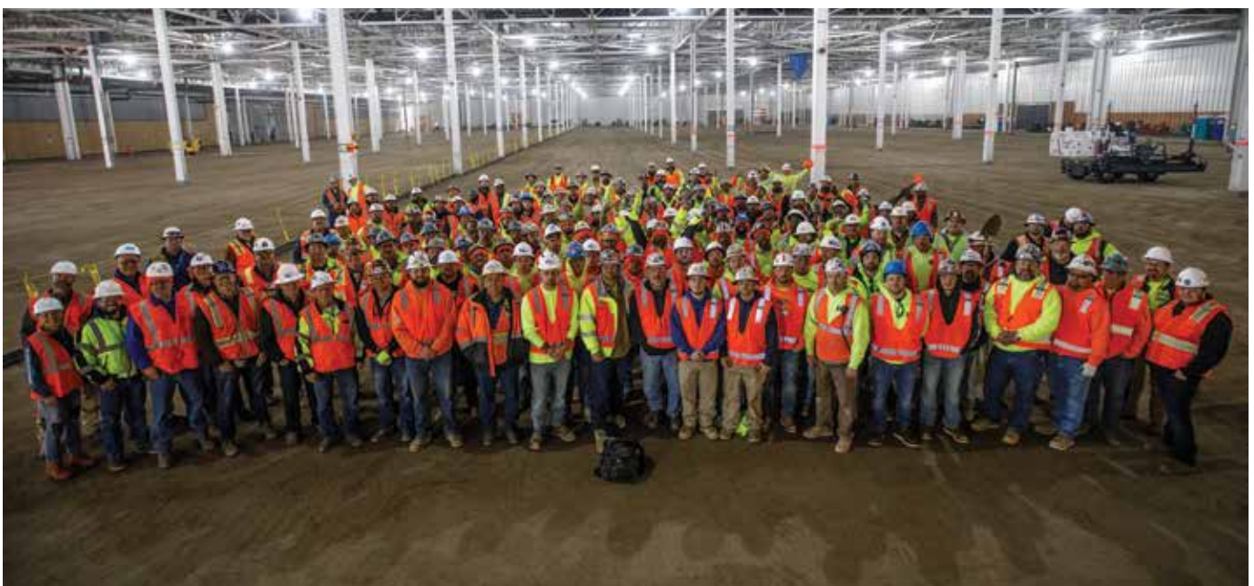
Prior to the placement of the Mega Slab, the crew assembled inside GM’s Arlington Assembly Plant, Arlington, TX (photo courtesy of Jon Humphrey)
