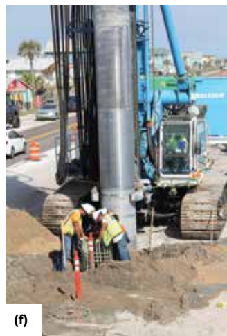
Fig. 6: A specialized drill rig was used to install the secant piles using the cased auger-cast method. The installation sequence comprised: (a) drilling; (b) soil removal and grouting; (c) GFRP cage lifting; (d) cage alignment; (e) cage insertion into the grout; and (f) final cage positioning
