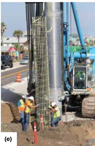
Fig. 6: A specialized drill rig was used to install the secant piles using the cased auger-cast method. The installation sequence comprised: (a) drilling; (b) soil removal and grouting; (c) GFRP cage lifting; (d) cage alignment; (e) cage insertion into the grout; and (f) final cage positioning
