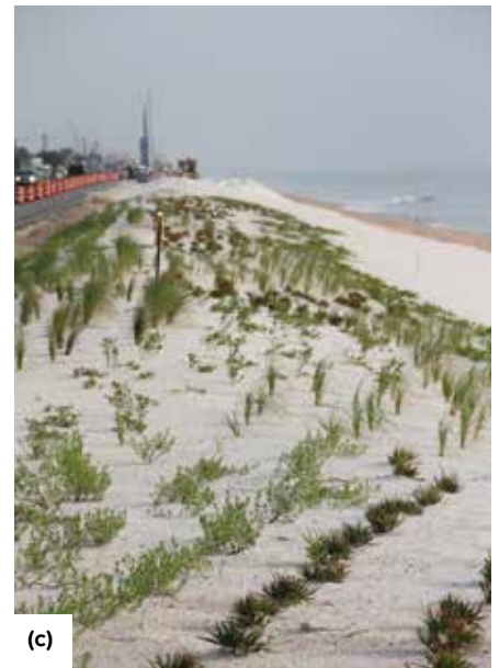
Fig. 7: After secant piles were installed: (a) the concrete guide wall was removed; (b) formwork and GFRP reinforcing bars were placed for the pile cap; and (c) a dune was constructed over the wall after the pile-cap concrete was placed and cured, and the pile-cap formwork was removed
